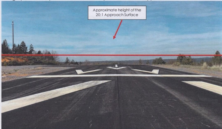
Photograph 2 - Trees penetrate the Runway 17 FAR Part 77 Approach and Transitional Surfaces.
