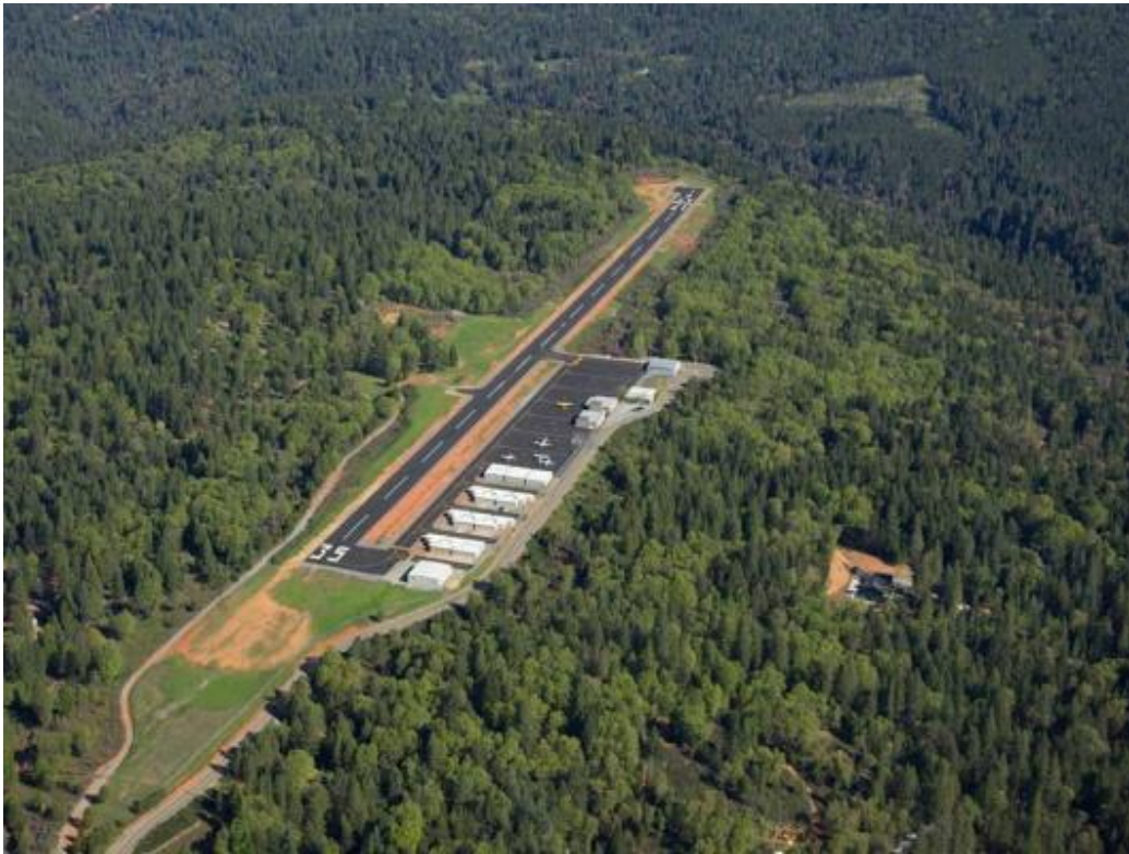
Figure 2 - Aerial view of Georgetown Airport circa 2002.
