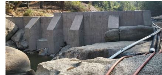
EID Outing dale dam after rehabilitation
