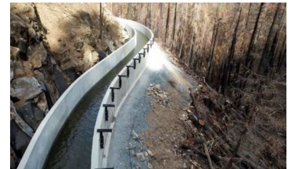
EID Flume 30 after repair
