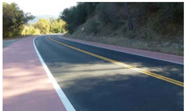
Figure 7-11: Example of red bike lanes on SR 49 in Coloma
