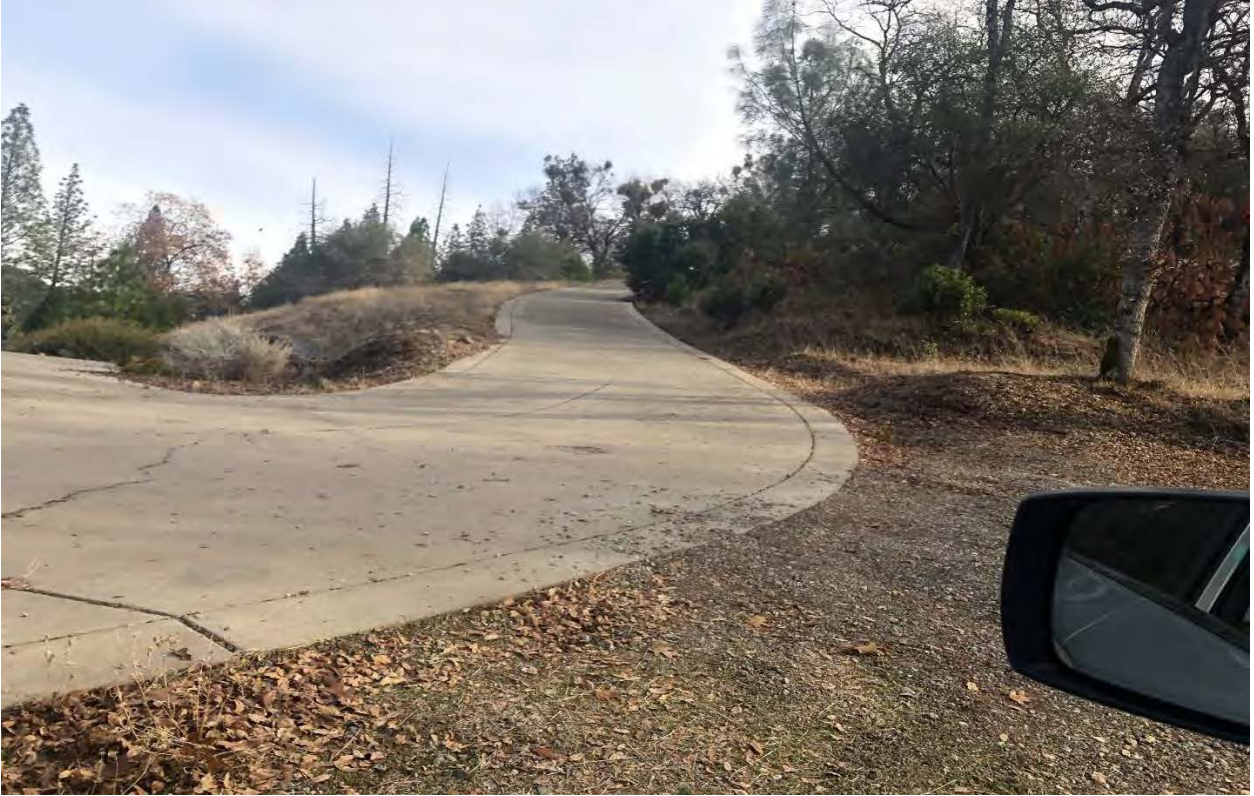
Photo 5: Paved access road entering into the parking area of the existing residence.
