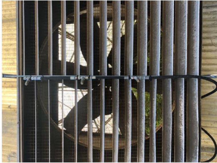
Figure 10 Details of Odor Control Misting Nozzles
