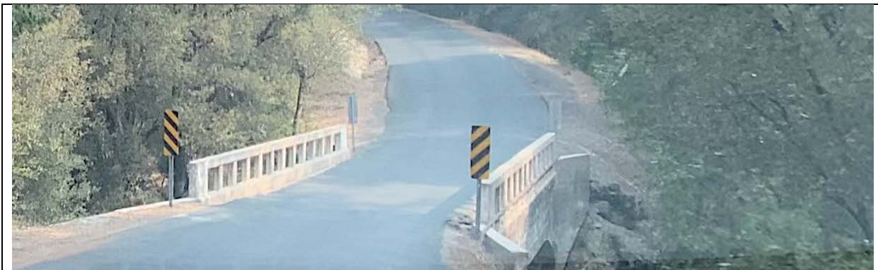
One lane bridge on Perry Creek Road looking east
