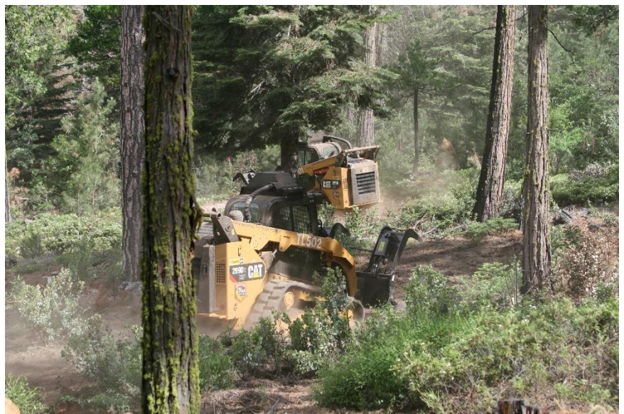
Mechanized management of vegetative fuels Photo courtesy of CAL FIRE
