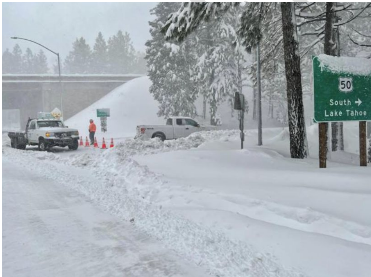
Figure 4-40 2023 Snowfall Impacting Roads Near South Lake Tahoe
