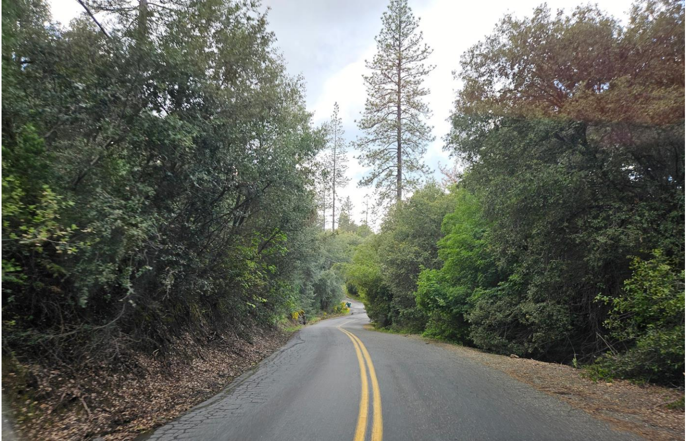
FIGURE 42: OUTINGDALE ROAD EXISTING CONDITIONS (APRIL 2024)
