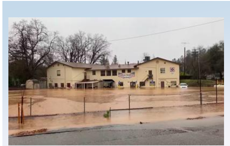
January 2023 Flooding of Veterans Memorial Building
