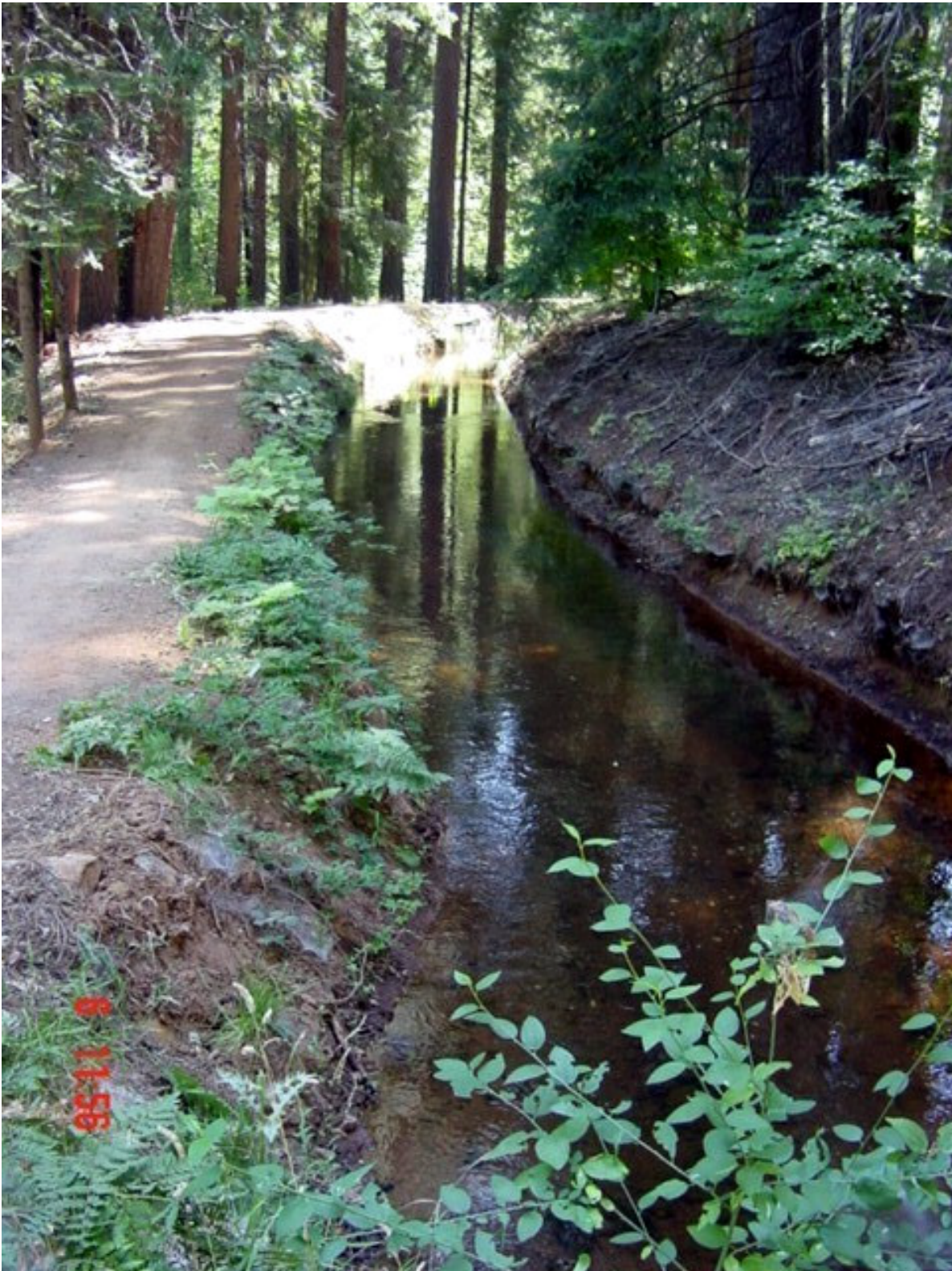
Sample of open ditch
