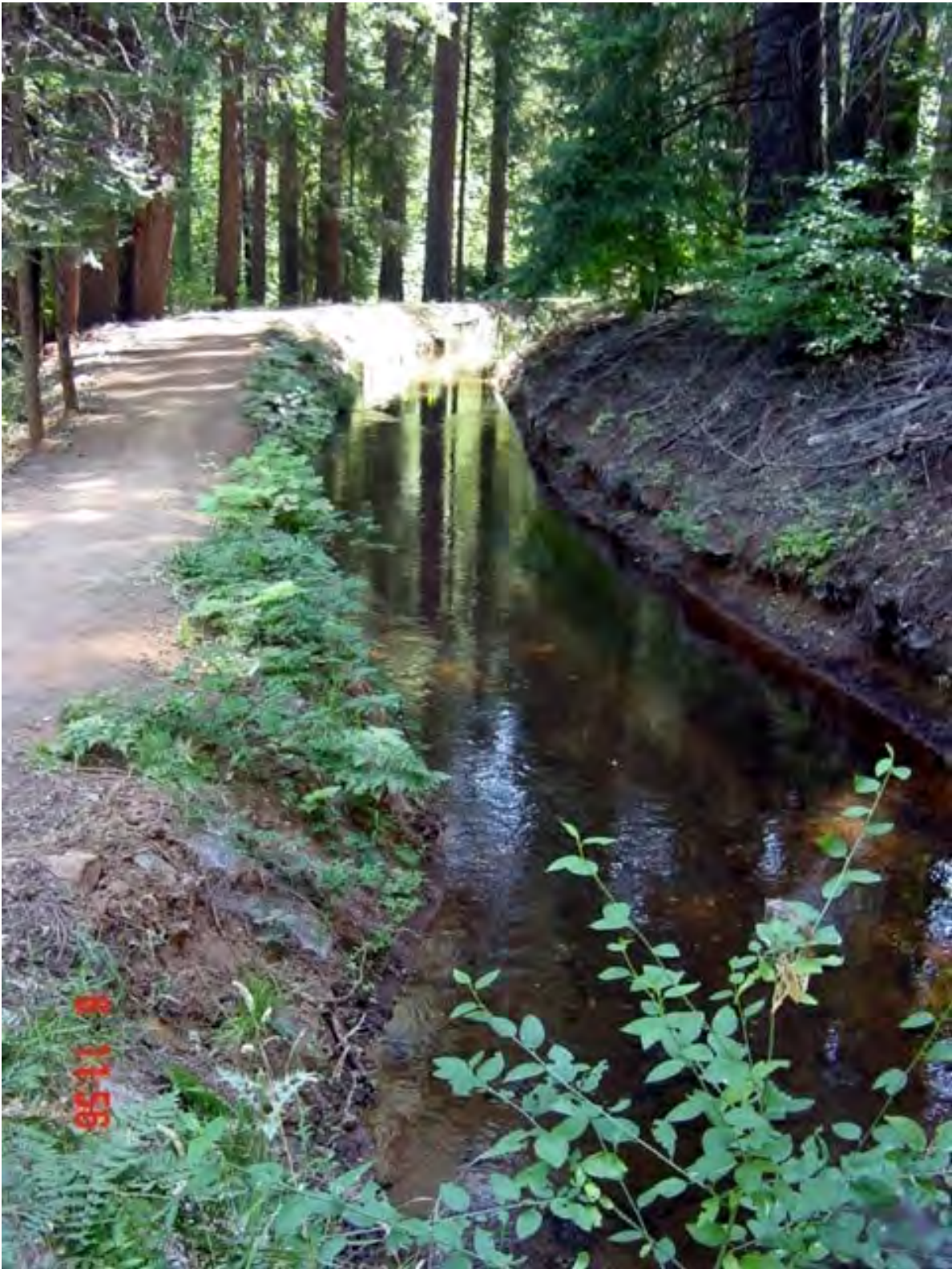
Sample of open ditch
