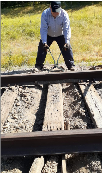
Rich Corbell has been volunteering with the EDWR for several years, and is always willing to help with whatever needs to be done – here he is getting his back into it working with a team replacing rotten ties – thanks Rich!
