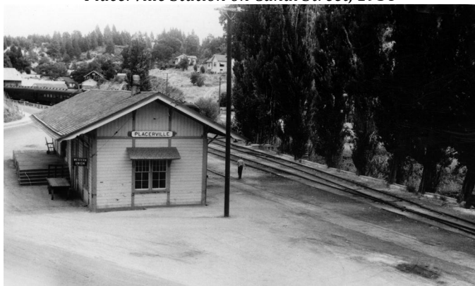
Placerville Station on Canal Street, 1938
