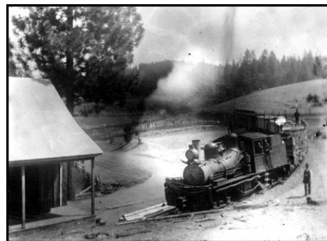
A Diamond & Caldor train hauling lumber pulls into Cole's Station on the way to the Diamond Springs Mill, c. 1920
