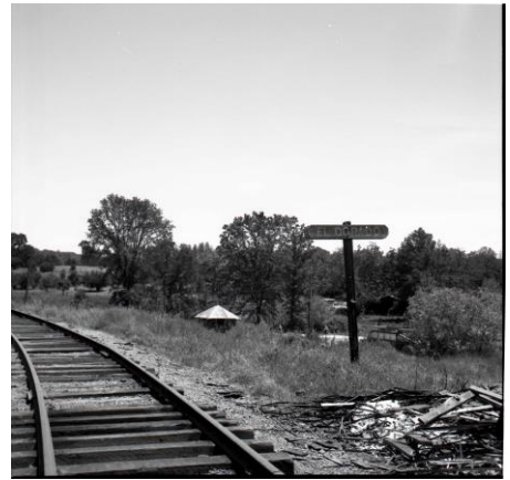
Site of the El Dorado Station after it was demolished
