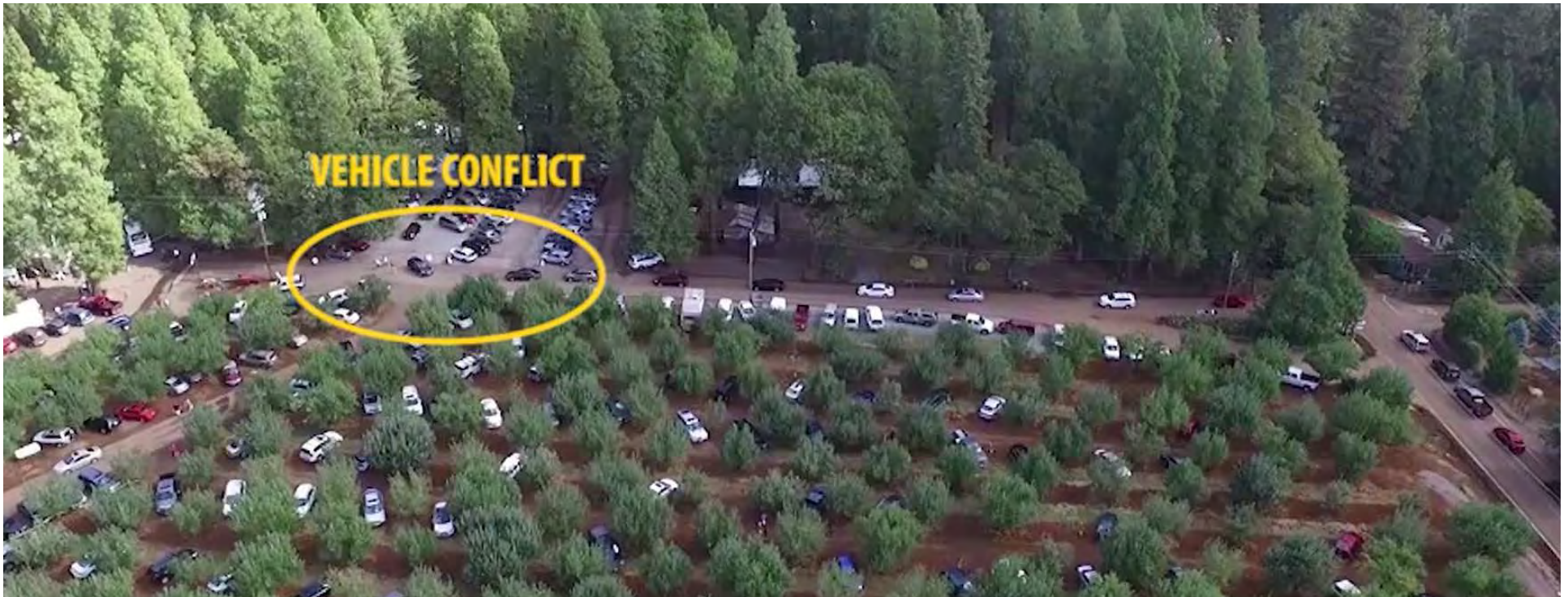
Figure 4: Aerial View of Carson Road/High Hill Ranch Road Area
