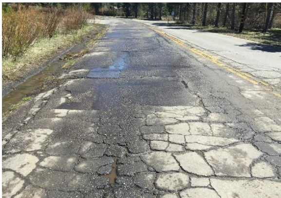
Figure S6. Pavement condition of Elks Club Drive before (left) and after (right) the installation of new asphalt overlay.
