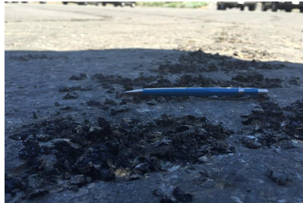
Figure S4. Pavement damage caused by snow plows (left) and rotary blades (right). A mechanical pencil was placed to show the scale of the damage.
