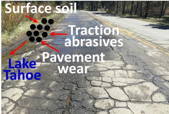
Before pavement rehabilitation
