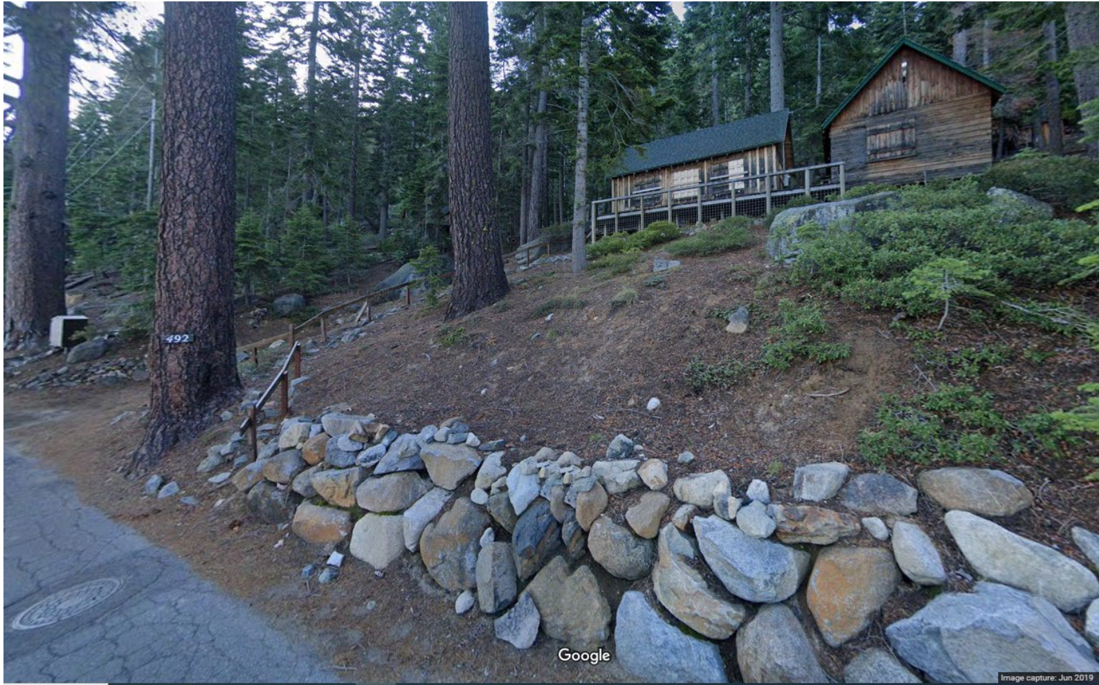
Existing rock retaining wall within roadway easement.
