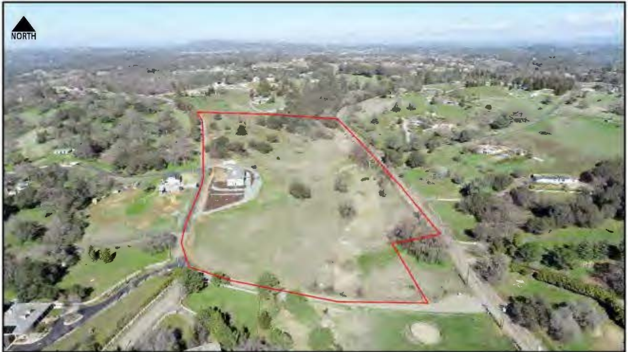
Looking north into the study area from Barnett Ranch Road. Photo Date 2-10-21
