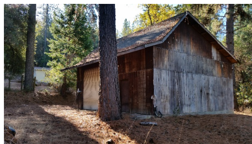
Two houses and one barn/garage on Parcel 1.
