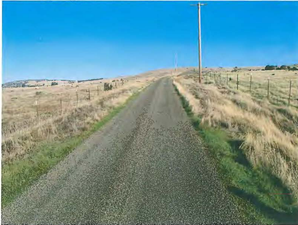
Photo 8. View looking north of the existing access road.
