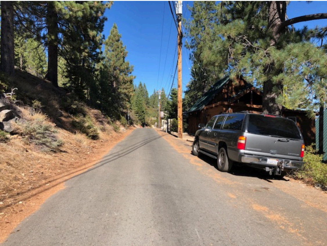
Meeks Bay Road looking north
