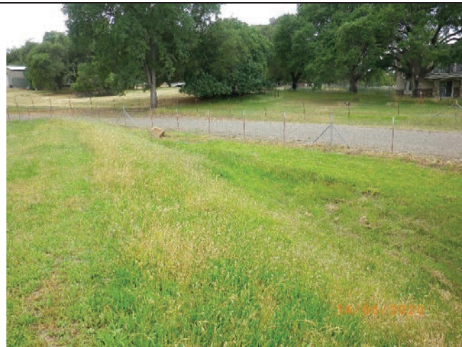
Photo 8. View of Channel 2 looking south, on the west side of the pond, from top of the berm. A portion of the berm around the pond is in foreground. 14 May 2020
