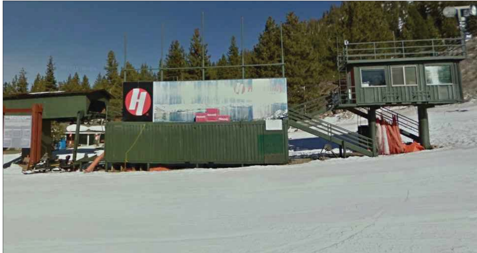
1 - PHOTO EXISTING CONDITION OF STRUCTURE
