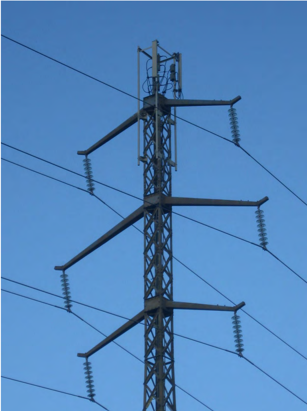
Photo showing the upper section of the electrical transmission tower
