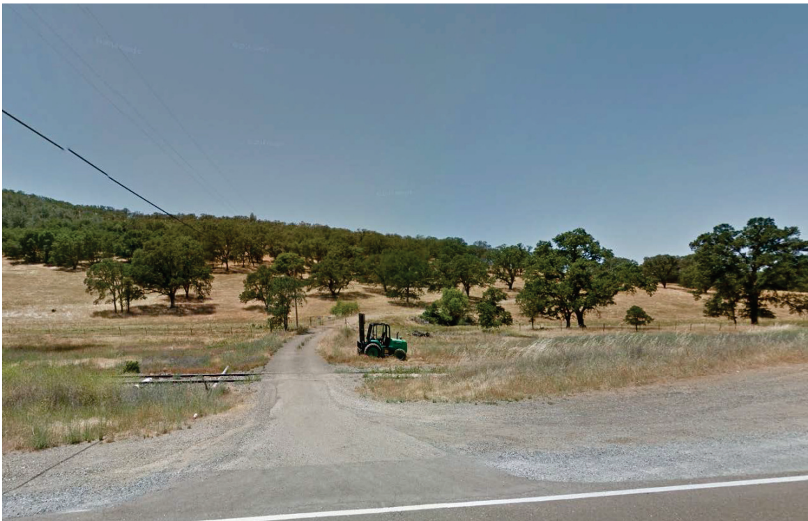
Driveway leading to American Tower site at Latrobe Road showing aggregate drive approach per Condition 7.
