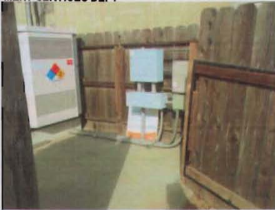
Entrance to Fenced Area
