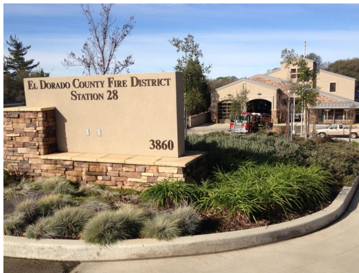
El Dorado County Fire Station # 28, Ponderosa Road, Shingle Springs
