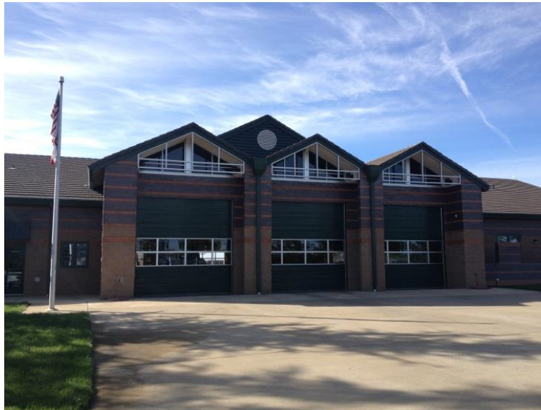
El Dorado Hills Fire Station # 86, Bass Lake Road, El Dorado Hills
