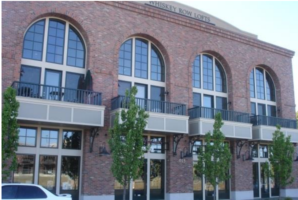
Sutter Court, Folsom (residential lofts above ground floor retail)
