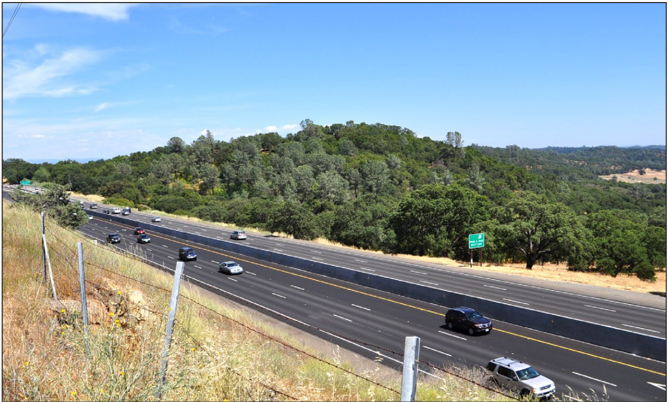
Photo 4: Looking southeast towards the project site from Country Club Drive, just north of US 50.
