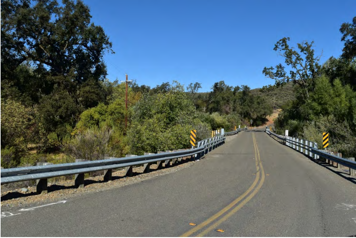
Looking North Northwest
