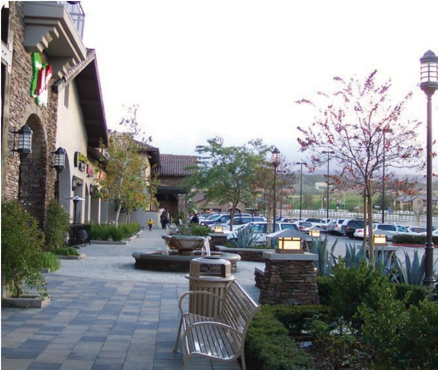
A landscape strip should be provided between a building and paved area
