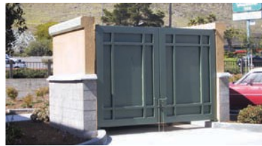
Trash enclosures should be screened
