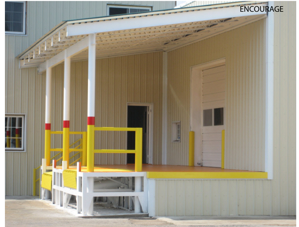
This loading dock's roof screens loading activities from the uses on the second level.
