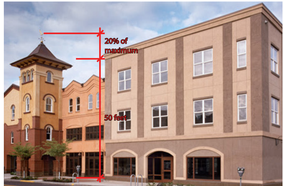
Spires, chimneys, and other projections can exceed the maximum building height by up to 20 percent.
