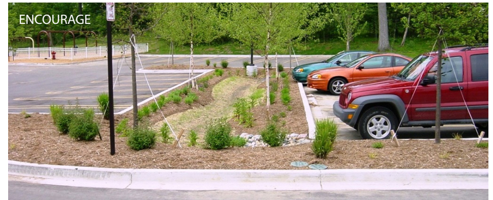
This parking lot features trees, landscaping, and a bioswale.
