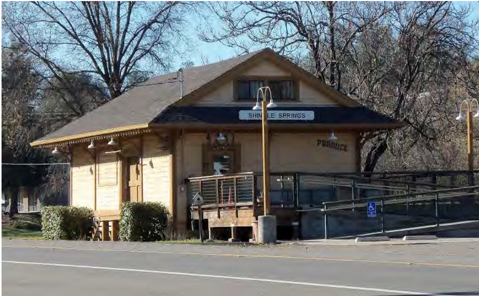
Figure 1: Shingle Springs Railroad Depot (single-story structure)
