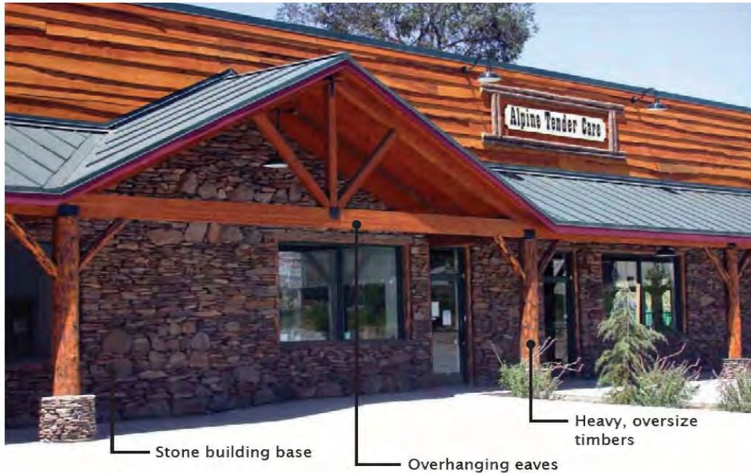
Figure 1. Mountain/lodge style commercial building
