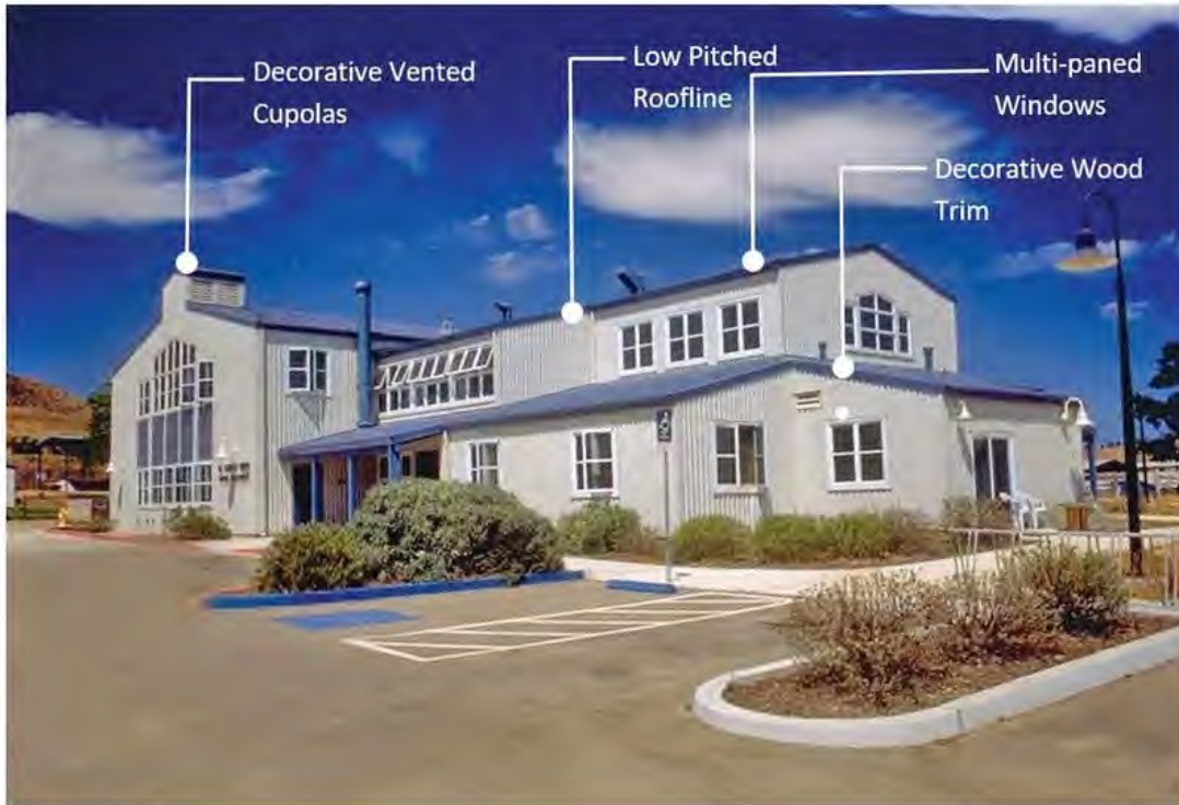
Figure 1. Mill / Agrarian Building
