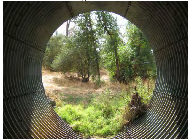
Inside culvert looking South
