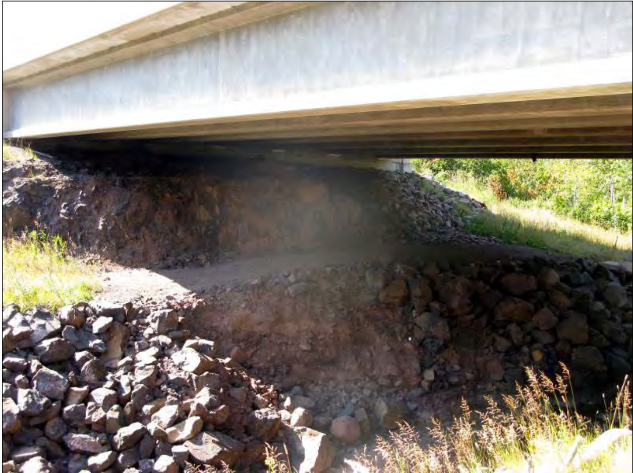
Figure 13. Level Walkway Added Under Existing Highway Bridge in Northern Minnesota to Facilitate Lynx Crossing
