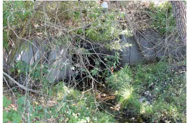
Close-up view of opening
