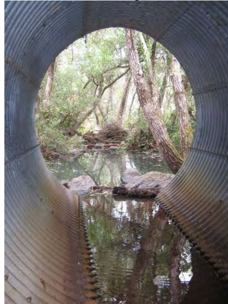
Inside culvert looking North
