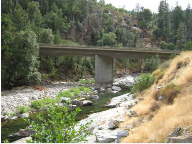
View under bridge from North
