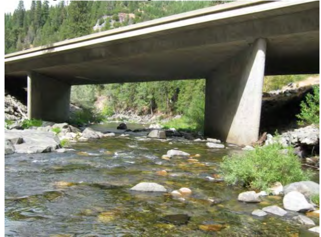
Looking N under bridge
