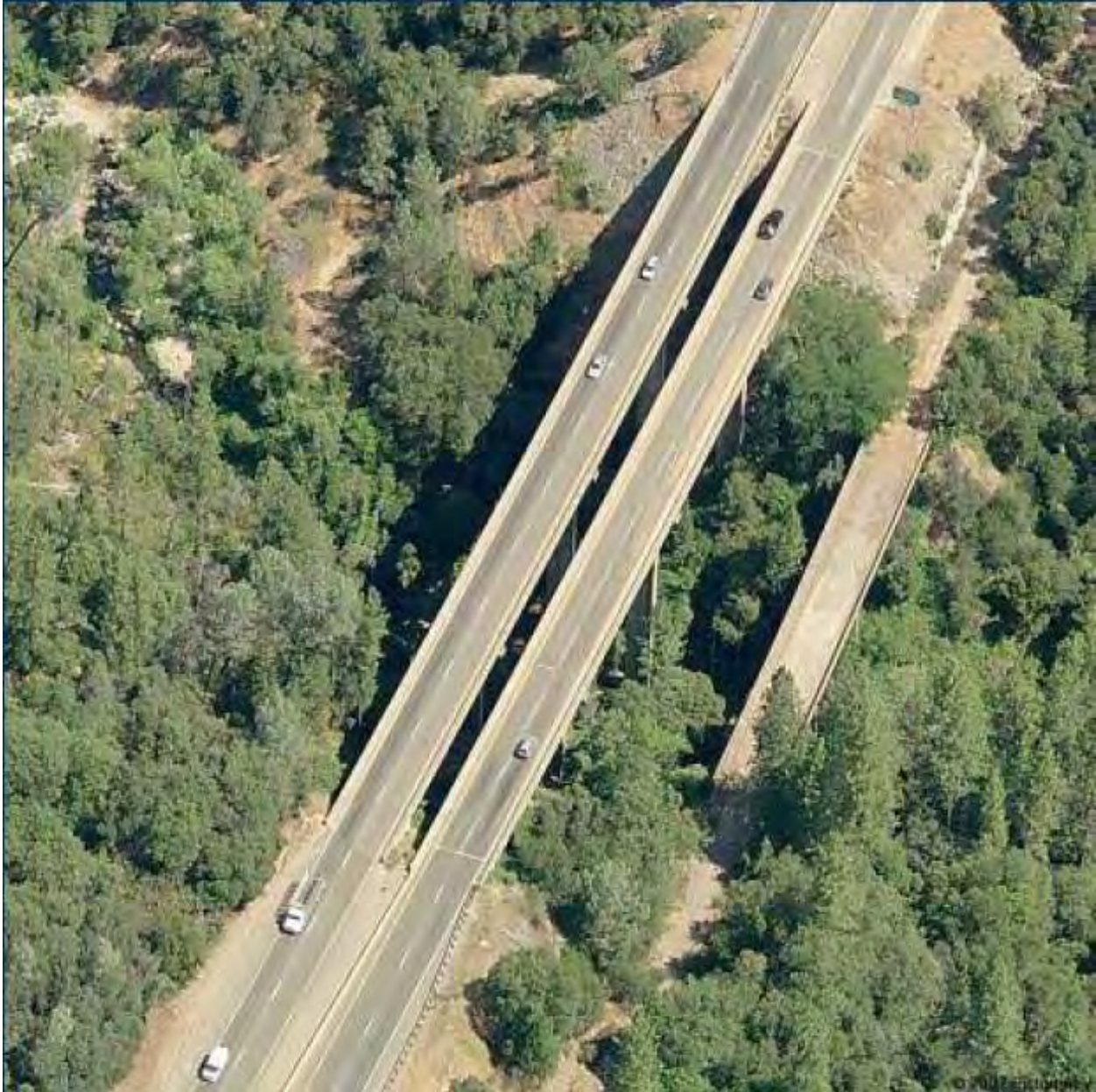
Figure 9. Weber Creek Under-Crossing
