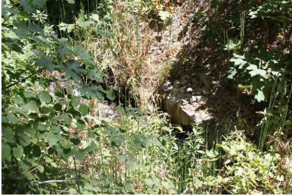
Close-up view of opening on North side
