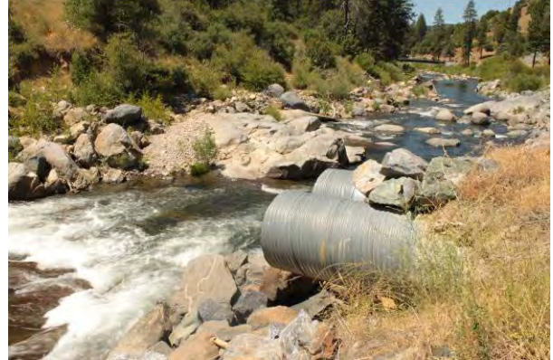
South side of culvert
