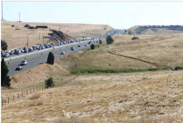
Westward medium view toward culvert
