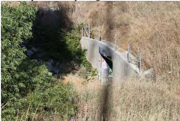
Close-up view of opening
