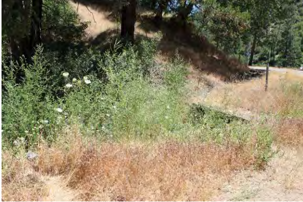
Medium view of opening from North side
