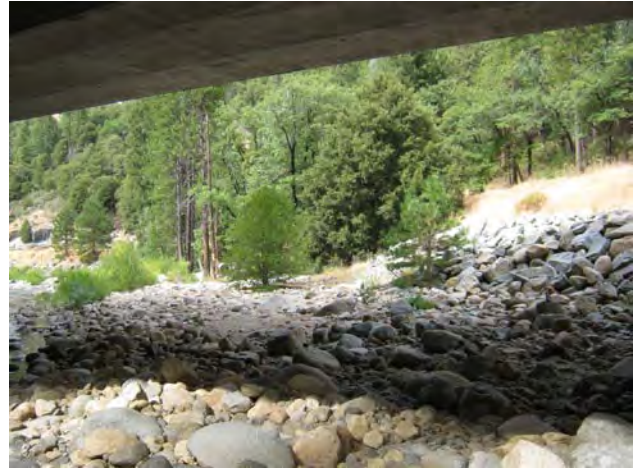
View North under bridge and adjacent vegetation
