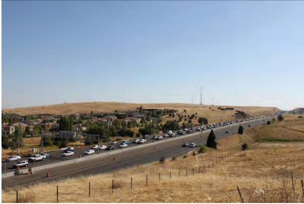
Westward landscape view toward culvert
