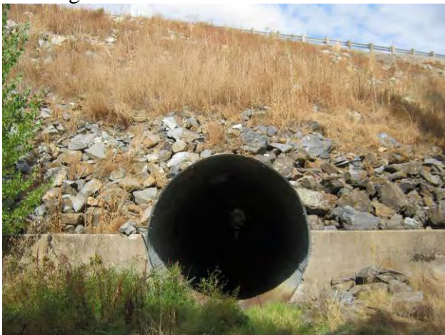
Looking North toward culvert
