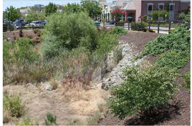
Westward close-up view second culvert
