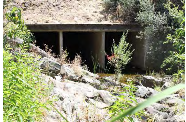
Close-up view of opening
