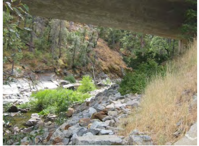
Rip-rap on West bank of under-crossing
