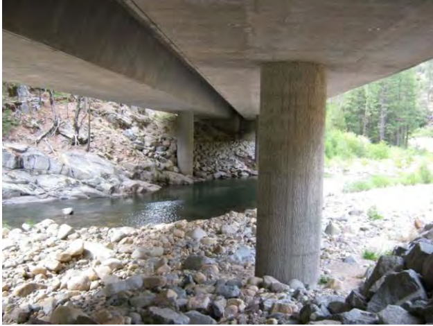
View under bridge looking West
