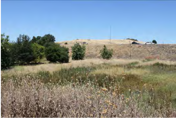
Westward medium view toward culvert
