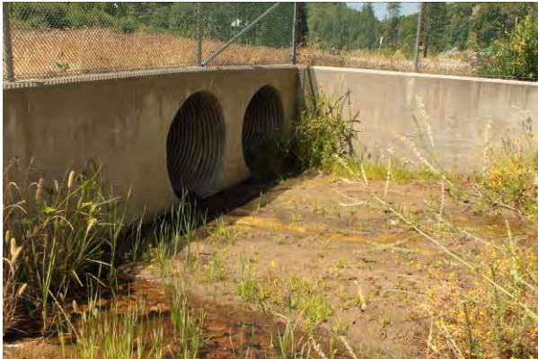
North side of culvert
