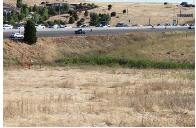
Westward closer view toward culvert
