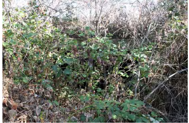
Close-up view of opening
