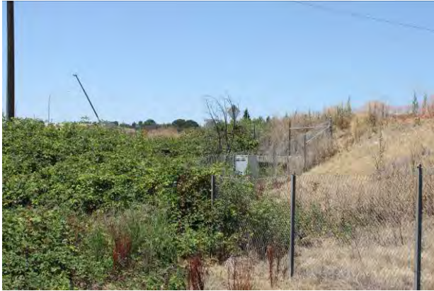
Westward close-up view highway culvert
