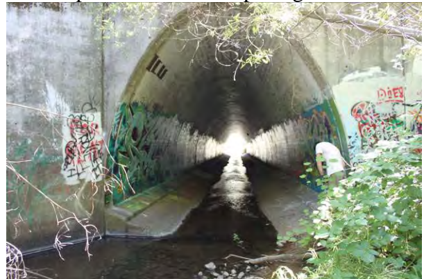
Close-up view of culvert opening
