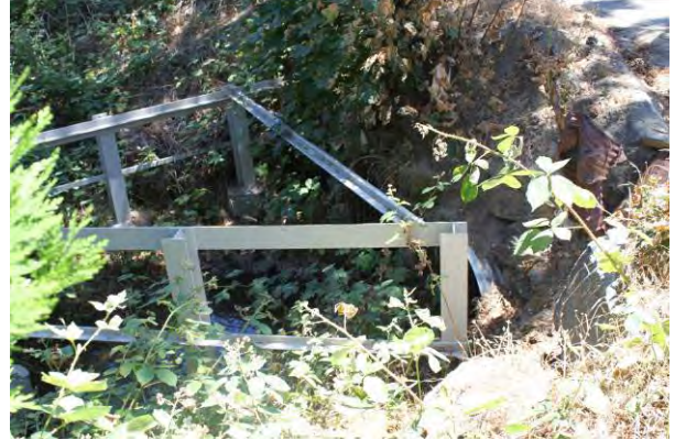
Close-up view North side
