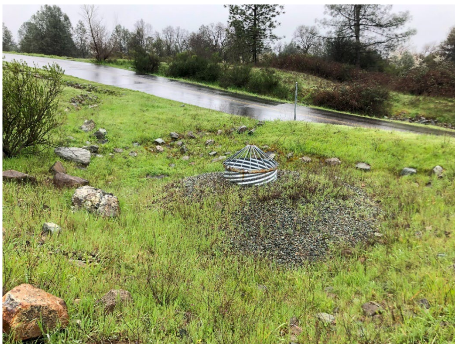
Photograph 8. South-facing view of storm water capture basin north of Rest Lane.
