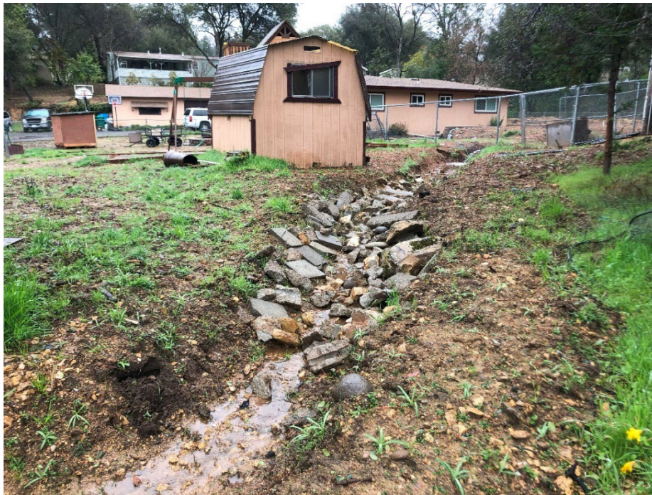
Photograph 9. Northeast-facing view of rock and earthen swale leading off private property in the northwest project area (water is from running hose near chain-link fence, not storm water).
