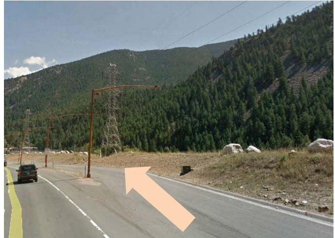
Figure 17: Separated Chain Up Example from I-70 in Idaho Springs, CO 21 (Aerial Image Source: Google Earth)
