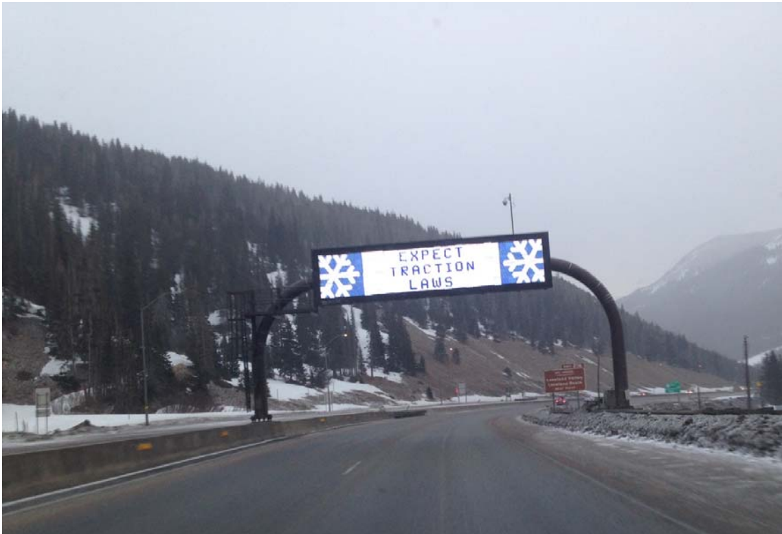
Figure 18: Permanent ITS Signs used in advance of Snow Storm on I-70 mountain corridor (Aerial Image Source: Google Earth)
