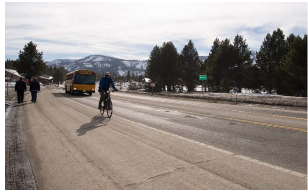
Large Right of Way leading to Santa Fe Rd Intersection. (Photo Source: Beryl)
