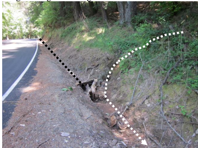
Photo 4. View southeast Ephemeral Channel 1 (dotted white line) confluence with UD-1 (dotted black line). Newtown Road on left. 12 June 2012.
