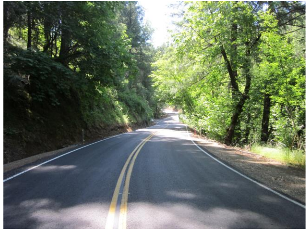
Photo 2. View west along Newtown Road from the eastern end of the BSA. Douglas fir forest on left; Oregon ash grove on right. 12 June 2012.
