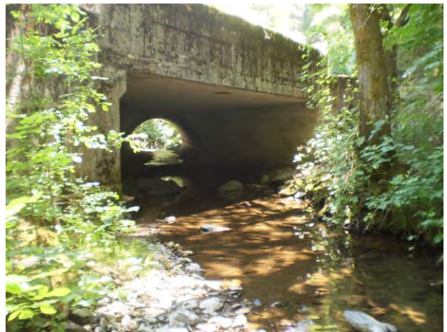
Photo 10. View west toward Newtown Road Bridge over South Fork Weber Creek. 12 June 2012.
