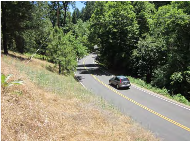
Photo 7. View east toward California annual grassland between Newtown Road (shown) and Paso Way (out of view on left). 12 June 2012.
