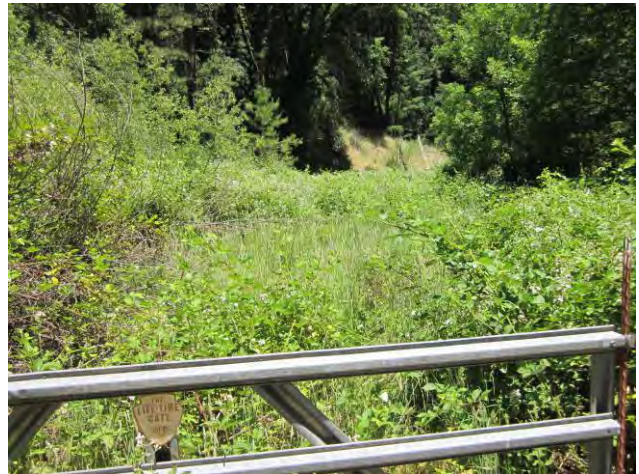
Photo 8. View north from the northeast corner of the bridge. Blackberry brambles shown. 12 June 2012.
