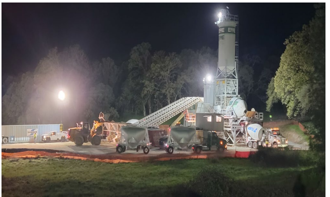
4/13/24 – Pier 3 Concrete Supply from Finnon Batch Plant
