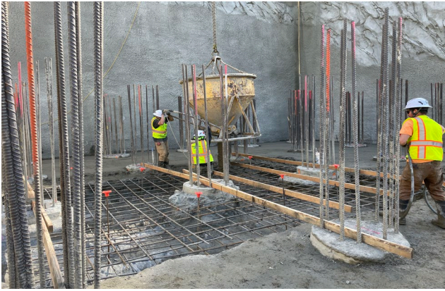
3/08/24 – Pier 2 Footing Rat Slab & VST Concrete Placement
