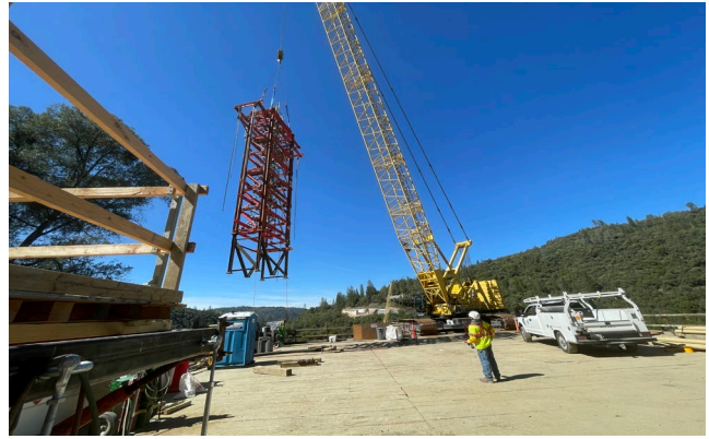
3/20/24 – Pier 2 VST Placement from Trestle
