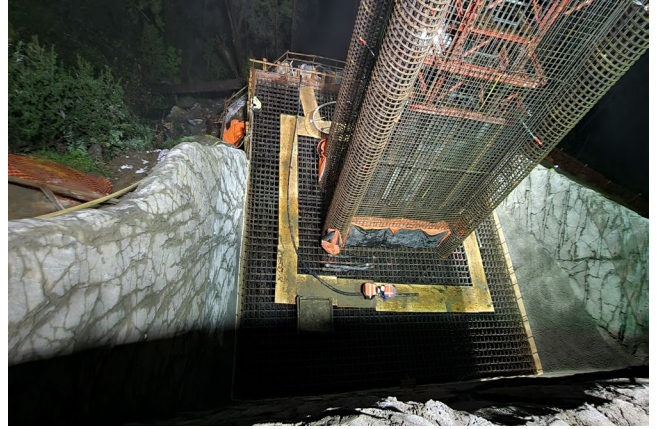
4/5/24 – Pier 2 Footing Concrete Placement (1,100 CY)
