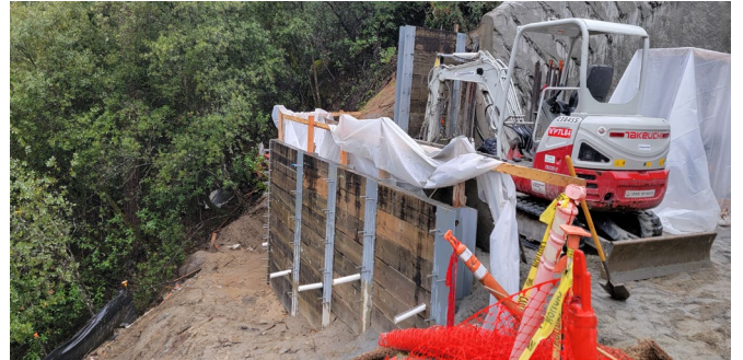
1/09/24 – Pier 3 Soldier Pile Walls
