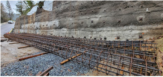
1/03/24 – Prefabricate & Stage Pier 2 CIDH Pile Cages
