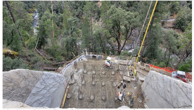
2/29/24 – Pier 2 Final CIDH & Soldier Pile Concrete Placement
