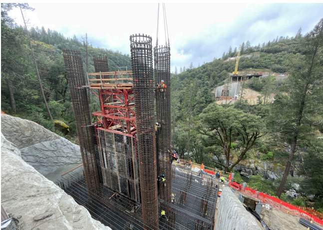
3/27/24 – Pier 2 Column Reinforcing Bar Cages Installation
