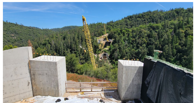
5/03/24 — View on Bridge Alignment from Abutment 4 (north)
