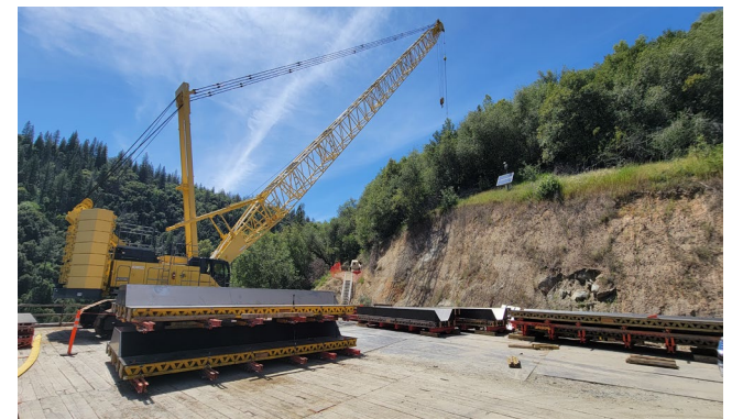
4/29/24 – Pier 3 Stage Lift 1 Exterior Forms at Trestle
