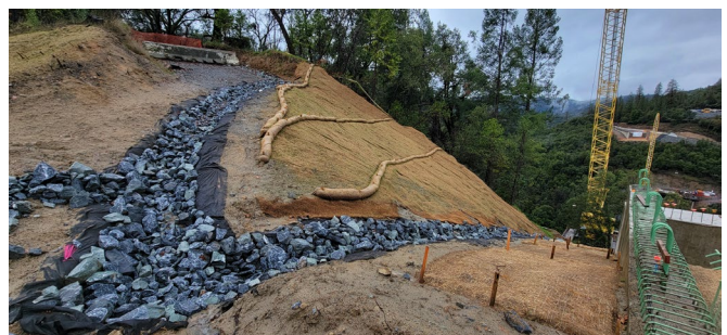
1/03/24 – Abutment 1 Erosion Control
