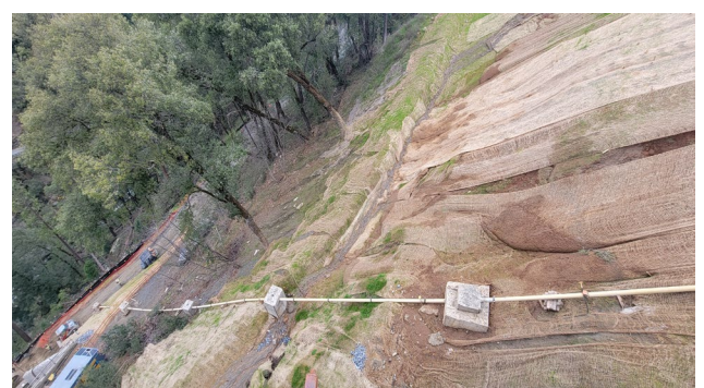
2/14/24 – Pier 2 Concrete Supply "Slick Line"
