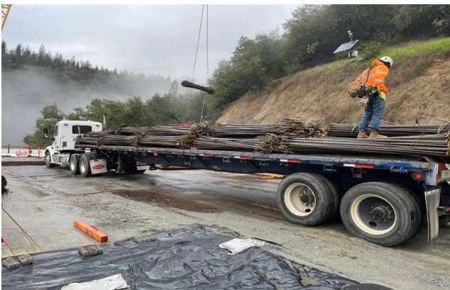
3/04-24 – Unload Pier 3 Footing Reinforcing Bar
