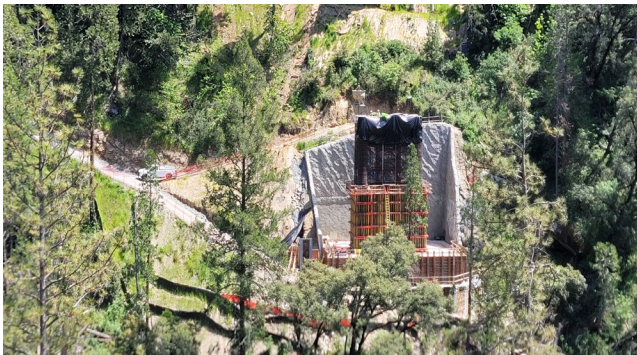
5/03/24 — Pier 2 Lift 1 Column Concrete Placement
