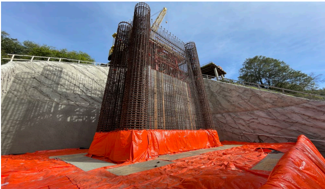
4/17/24 – Pier 3 Concrete Thermal Cure
