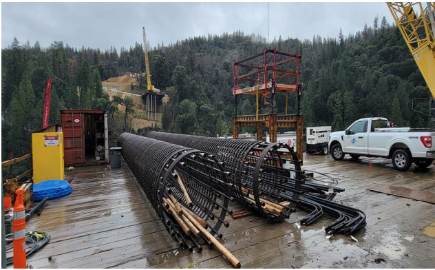
2/02/24 – Prefabricated Pier 3 Column Reinforcement
