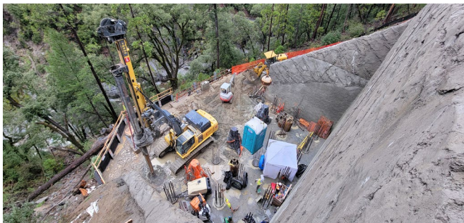
1/03/24 – Continued Installing Pier 2 CIDH Piles
