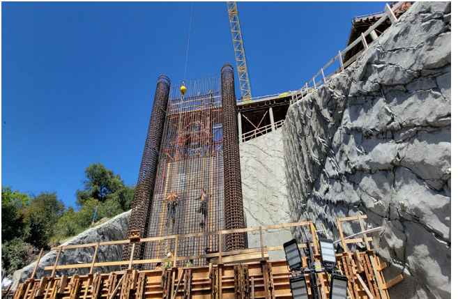
4/11/24 – Pier 3 Shear Wall Reinforcing Steel Installation
