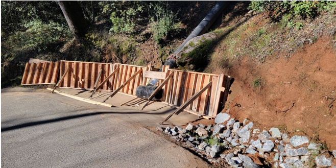
1/05/24 – DS-5 Outfall Wall Construction
