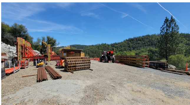
5/03/24 —Pre-assembly & Staging of Pier 3 Work Platforms
