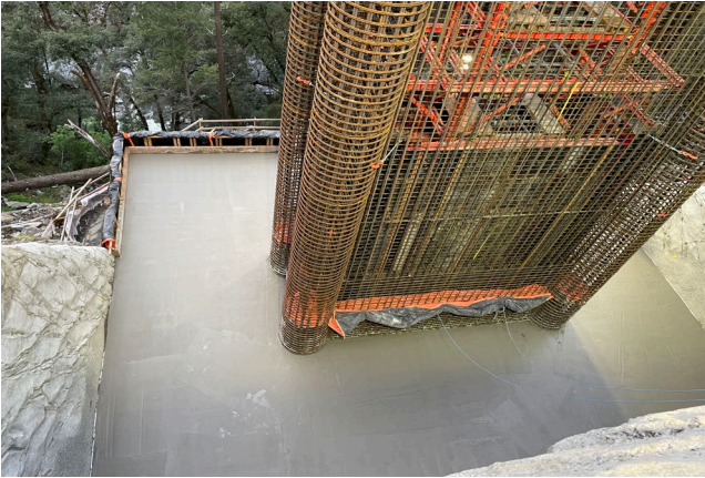
4/6/24 – Pier 2 Footing Concrete Placement Complete
