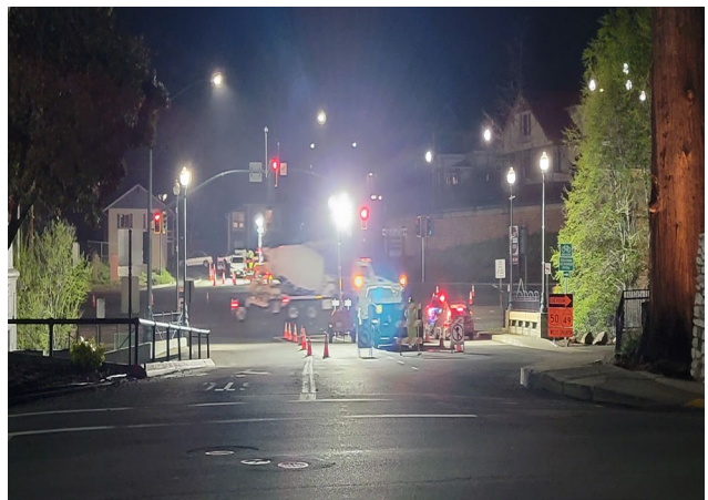
4/5/24 – Hwy 50 “Trip to Green” for Pier 2 Concrete Haul
