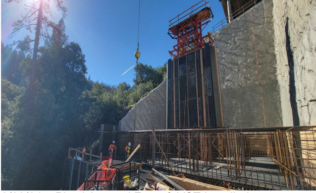
2/28/24 – Pier 3 Internal Form & VST Installed
