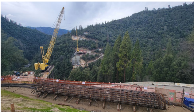
2/14/24 – Prefabricated Pier 2 Column Reinforcement
