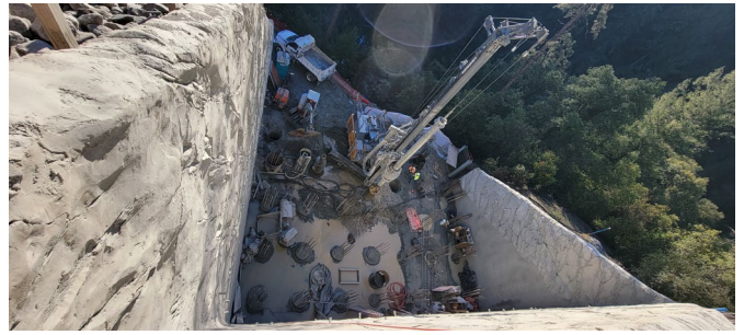
1/05/24 – Continued Installing Pier 3 CIDH Piles
