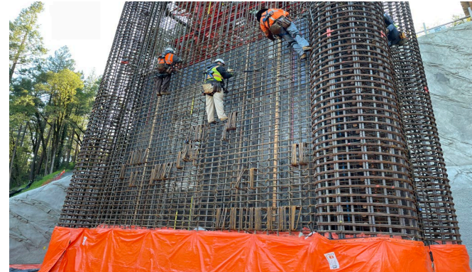
4/17/24 – Pier 2 Install Shear Wall Reinforcement Hairpins
