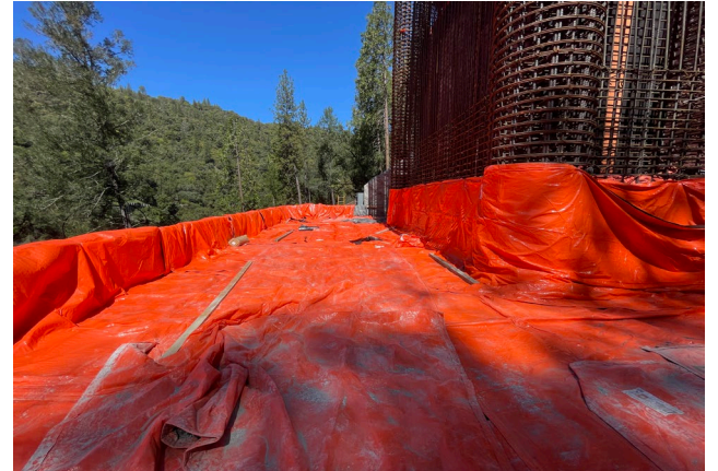
4/6/24 – Pier 2 Footing Concrete Thermal Cure
