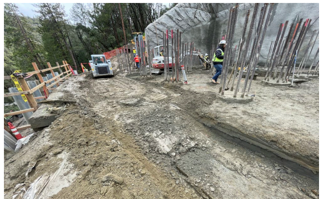
3/05/24 – Pier 2 Footing Subgrade & VST Footing Excavation
