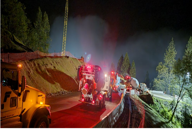
4/5/24 – Pier 2 Concrete Truck Staging
