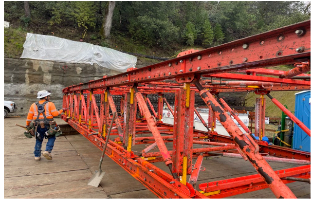
3/12/24 – Pier 2 VST Construction & Staging on Trestle
