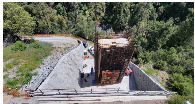
5/03/24 — Pier 3 Begin Installation of Lift 1 Exterior Form Panels
