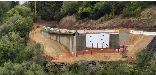
1/22/24 – Abutment 4 Erosion Control
