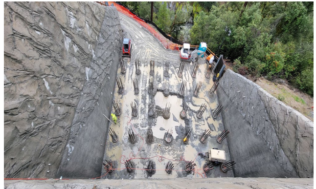
2/02/24 – Pier 3 CIDH Piles & VST Footing Exc.
