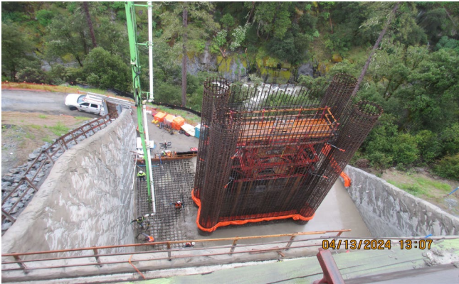
4/13/24 – Pier 3 Footing Concrete Placement
