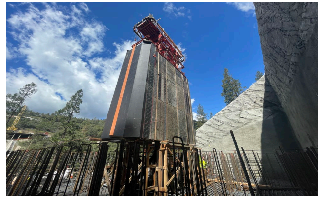
3/25/24 – Pier 2 Install Interior Column Form Panels on VST
