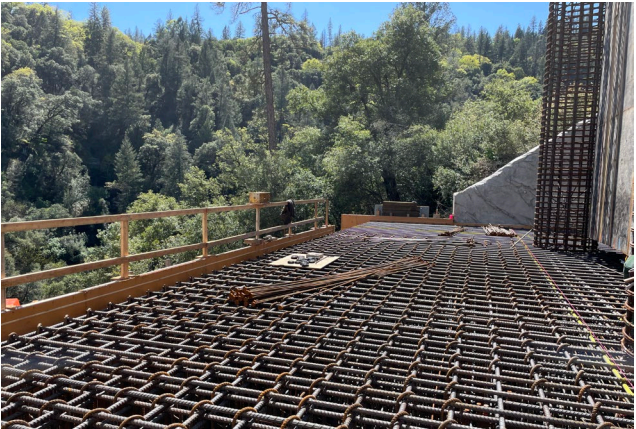
4/09/24 – Pier 3 Top Mat Reinforcement Complete
