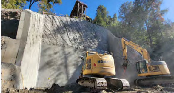
9/27/23 – Pier 2 Shotcrete Completed / Start Footing Prep.
