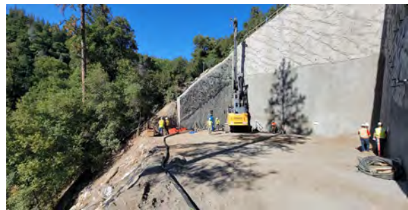
10/02/23 – Start Drilling First Pier 3 CIDH Pile
