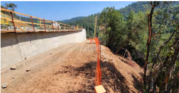
8/31/23 – Abutment 4 RW 4 Completed & Structure Backfill
