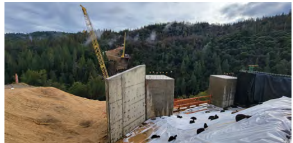
1/03/24 — Abutment 4 Erosion Control Measures
