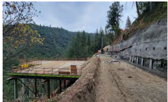
9/01/23 – Progress P2 Trestle Access Temp. Soil Nail Wall
