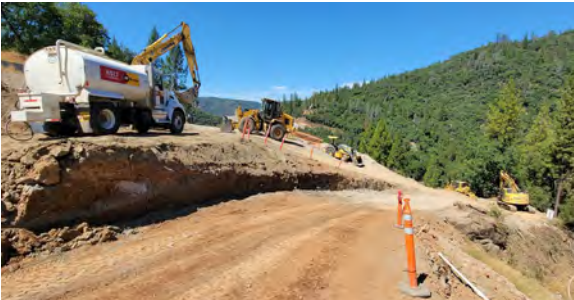
9/08/23 – Abutment 1 Approach Fill, P2 Access Road
