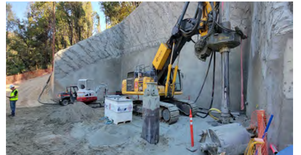
10/19/23 – Pier 2 CIDH Pile Drilling
