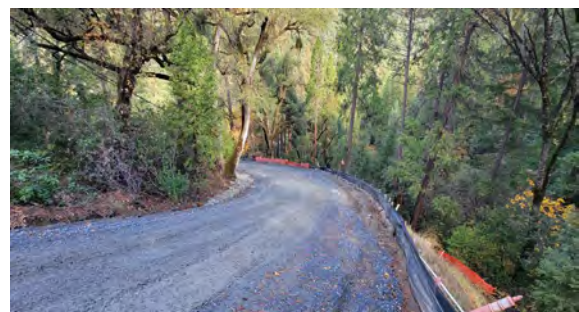
11/17/23 – Pier 2 Rocked Access & Ditch, Silt Fence
