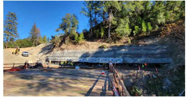
9/27/23 – Progress P2 Trestle Access Temp. Soil Nail Wall
