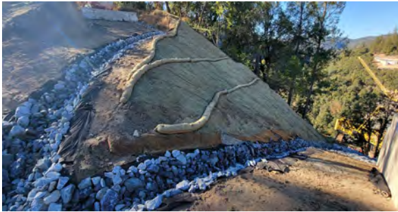
11/17/23 – Abutment 1 Slope Protection & Rock Ditches
