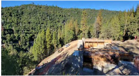
9/27/23 – Abutment 1 Retaining Walls Formed
