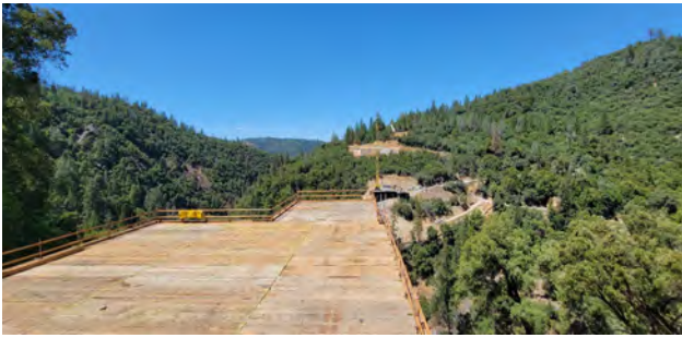
8/17/23 – South Pier 2 Trestle Looking North
