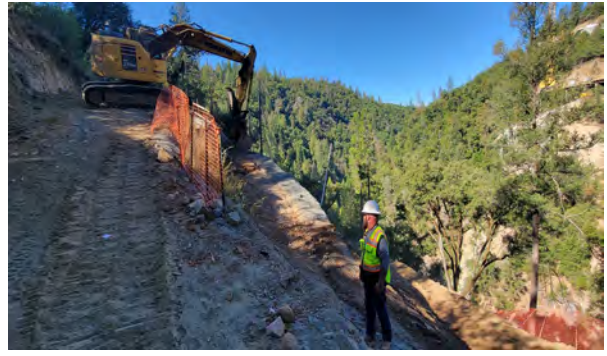
10/02/23 – Pier 2 East Rock Lined Ditch Excavation
