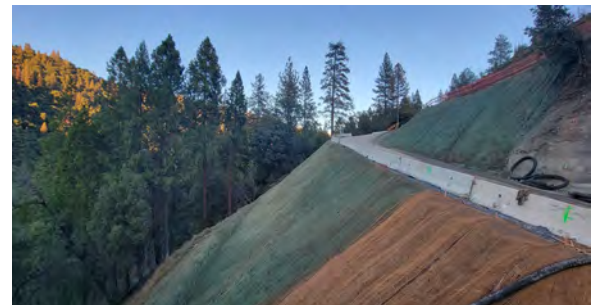
10/26/23 – Pier 2 Trestle Access Hydroseed #1
