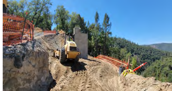
9/08/23 – Abutment 1 Structure Backfill
