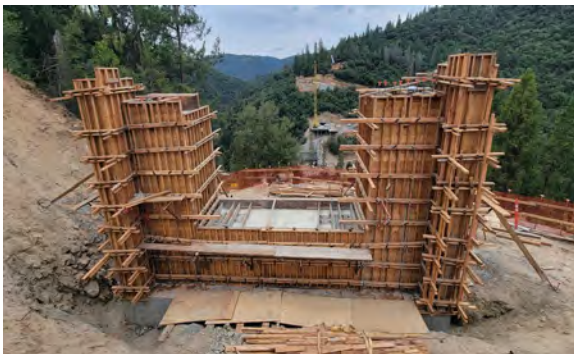
9/01/23 – Abutment 1 Footing & Stem Concrete Placed
