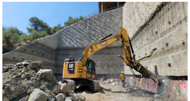
8/31/23 – Pier 3 Hard Rock Structure Excavation – Last Lift
