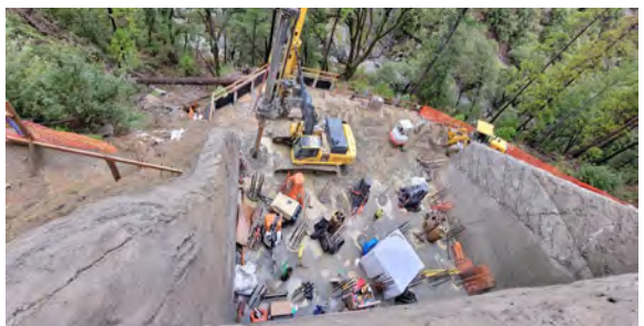
1/03/24 — Pier 2 Commence Drilling 13 Remaining Piles
