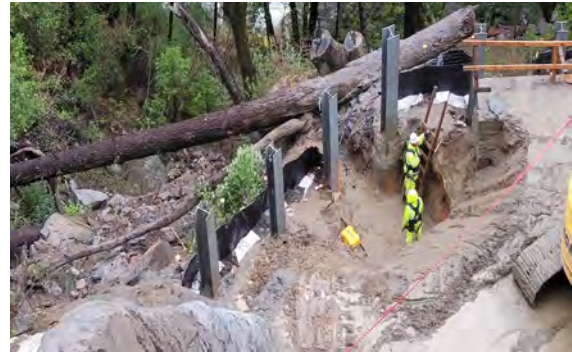
12/20/23 – Pier 2 Soldier Piles & DS-7 Installation
