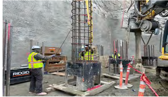
11/27/23 – Pier 3 Set CIDH Pile Cage
