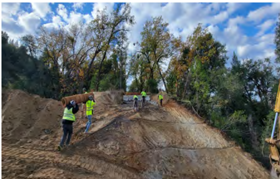
11/17/23 – Abutment 1 Slope Erosion Control Installation
