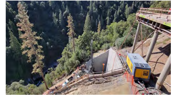
10/13/23 – Pier 3 First CIDH Pile Concrete Placement
