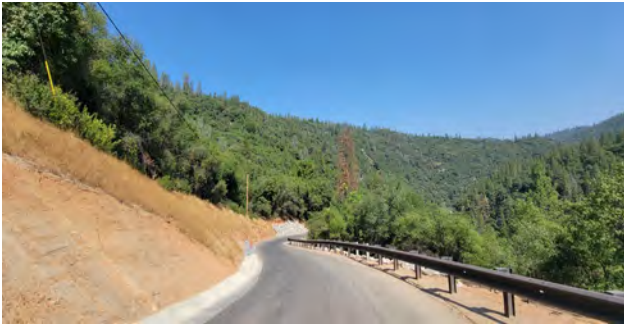
8/08/23 – North Guardrail, Ditches, RSP Slopes Completed
