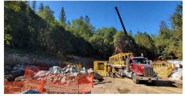
10/02/23 – Unload Pier 2 Crane Boom Sections
