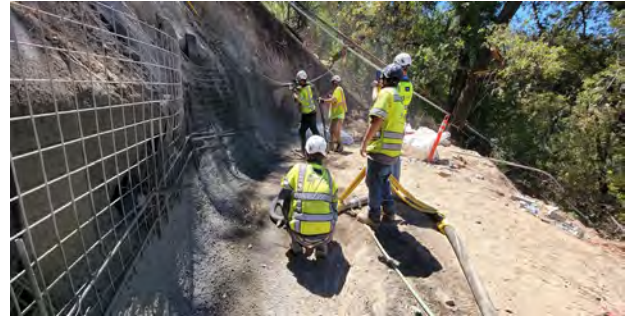
8/17/23 – P2 Trestle Access Temp. Soil Nail Shotcrete Lift 1
