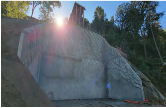
10/02/23 – Pier 2 Ready for CIDH Piles Installation
