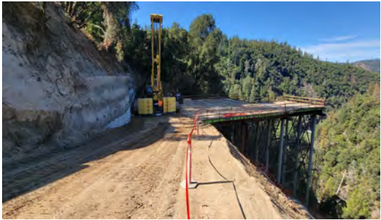
10/02/23 – Mobilize Crane to Pier 2 Trestle & Assemble
