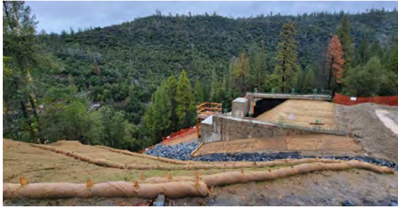
1/03/24 — Abutment 1 Erosion Control Measures
