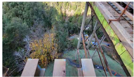
11/17/23 – Erosion Control Under Pier 2 Trestle
