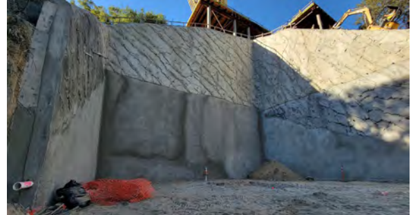
9/27/23 – Pier 3 Shotcrete Completed / Start Footing Prep.
