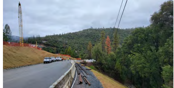
1/03/24 — Pier 2 Access Erosion Control Measures
