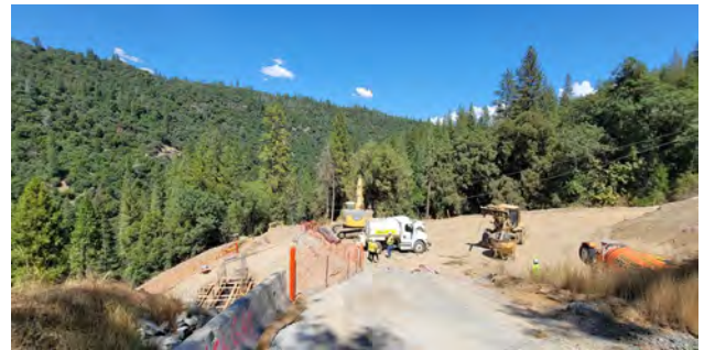
8/17/23 – Abutment 1 Footing Concrete Placement
