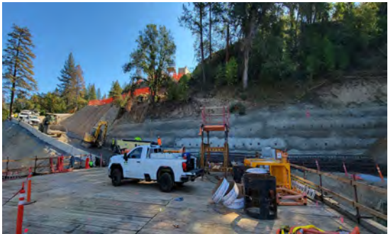
10/13/23 – Access Road Paved and Heavy Use
