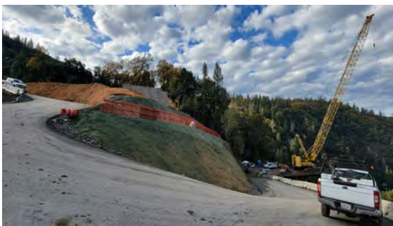
11/17/23 – Paved Pier 2 Access, Rock Lined Ditches
