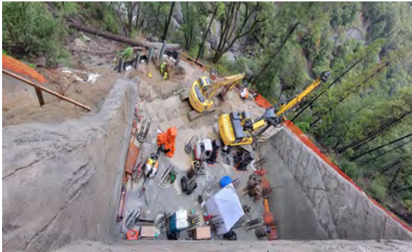
12/20/23 – Pier 2 CIDH Piles 21 of 35 Piles Completed
