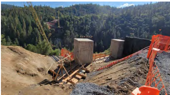
10/24/23 – Abutment 4 East Wingwall Construction
