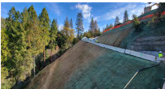
11/17/23 – Trestle Access Blanket & Hydroseed #2
