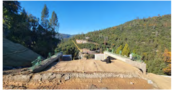
11/17/23 – Abutment 1 Looking North
