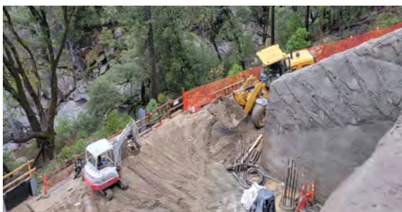
1/04/24 — Pier 2 Load & Haul Out Drill Spoils
