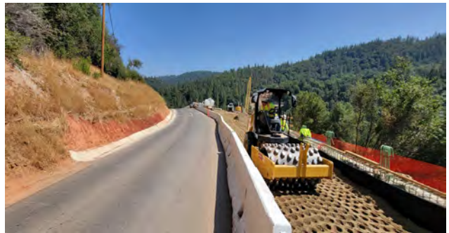
8/31/23 – Abutment 4 RW 4 Completed & Structure Backfill
