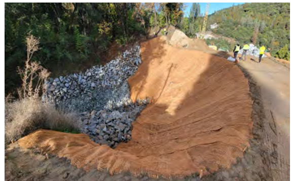
11/17/23 – DS-3 Inlet RSP Armoring & EC Blanket
