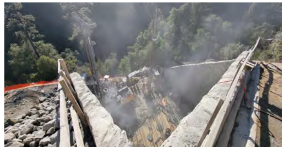
1/05/24 — Pier 3 Drilling & Placing CIDH Pile Rebar
