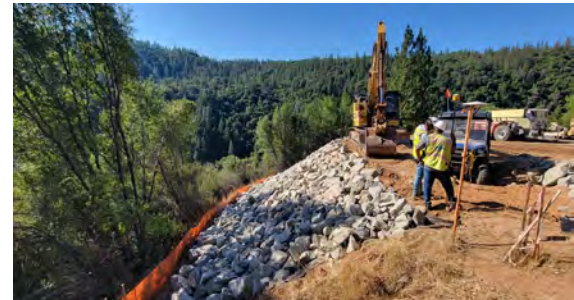
9/18/23 – RSP Slope Armoring at BLM Embankment
