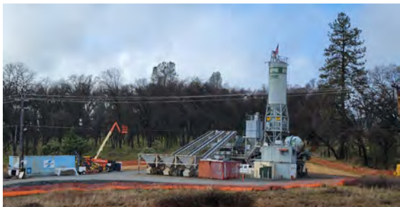
1/03/24 — Batch Plant Erosion Control Measures
