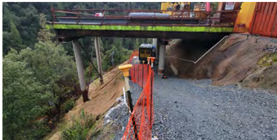
1/03/24 — Pier 3 Trestle Erosion Control Measures
