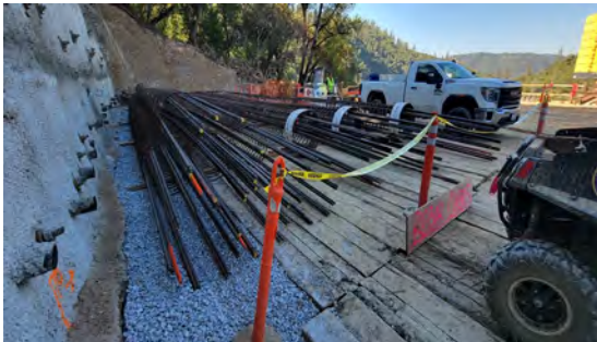
10/19/23 – Pier 2 CIDH Rebar Cage Fabrication
