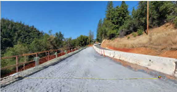
9/18/23 – Base Grade Abutment 4 Approach
