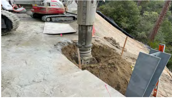
11/17/23 – Pier 3 Soldier Pile Wall Pile Drilling
