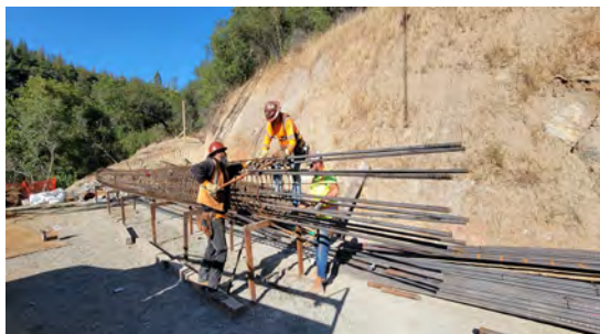
10/02/23 – Fabricate First Pier 3 CIDH Rebar Cage
