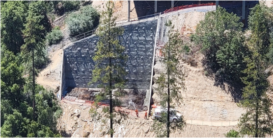
7/21/23 - Pier Row 3 Hard Rock Blasting Preparation
