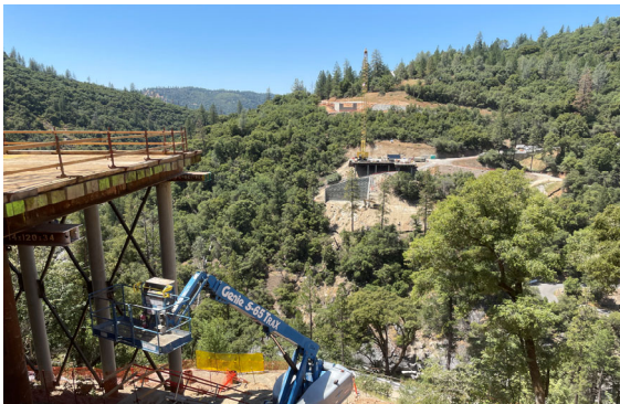
7/05/23 – South Trestle Bracing Installation
