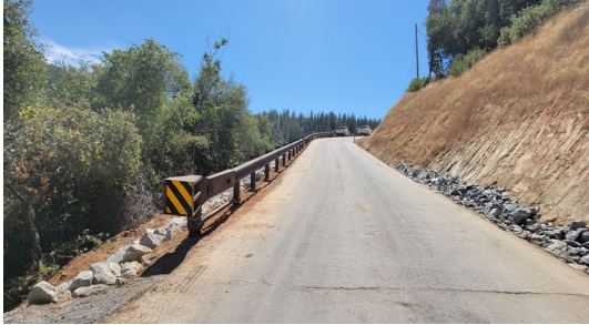
8/01/23 — North Metal Guardrail System Complete
