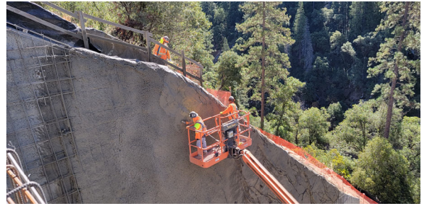
8/01/23 — Pier 3 Rows 13-5 Architectural Shotcrete
