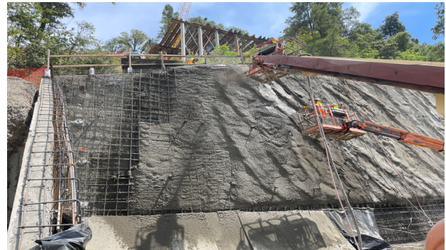
6/28/23 - Pier 2 Rows 11-6 RW Architectural Shotcrete
