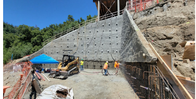
6/13/23 - Pier 3 Rows 6 RW Progress / Shotcrete
