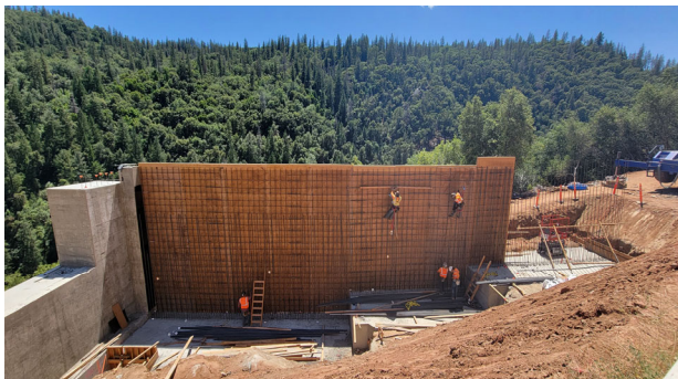
6/19/23 – Abutment 4 RW 4 Stage 1 Stem Rebar Installation
