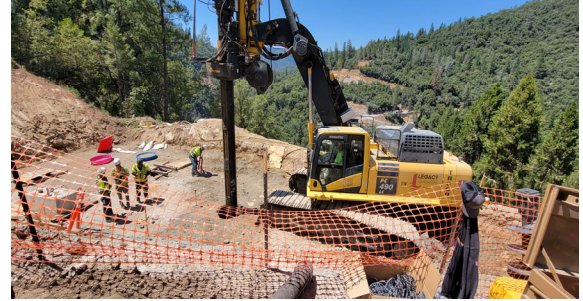
7/19/23 – Abutment 1 Foundation CIDH Pile Installation
