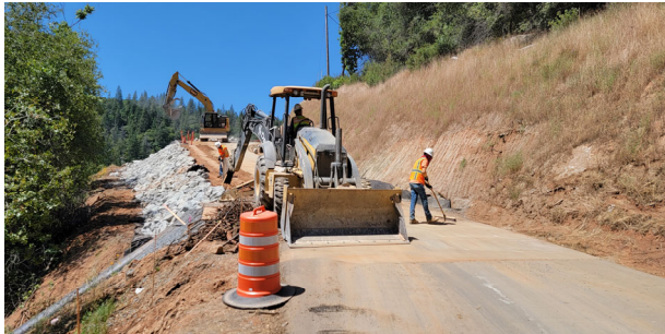
6/13/23 – North Rock Slope Protection Installation
