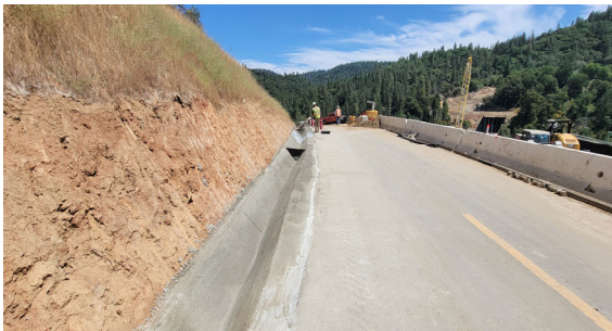
8/03/23 — North Concrete Lined Ditch Progress
