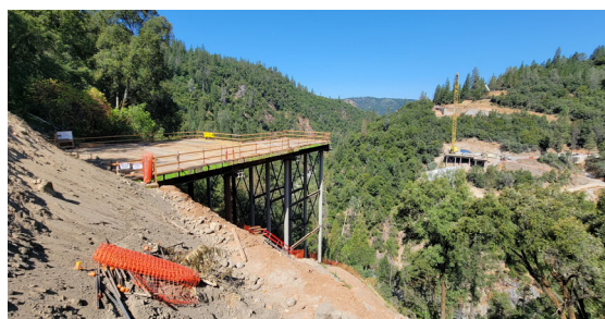
8/04/23 — Pier 2 Trestle Complete Looking North
