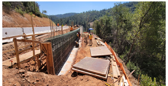
8/04/23 — RW 4 Stage 3 Stem Rebar Installation
