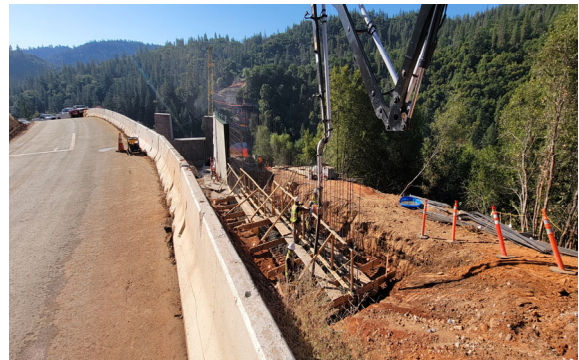
7/06/23 - Abutment 4 RW 4 Stage 2 Footing Pour
