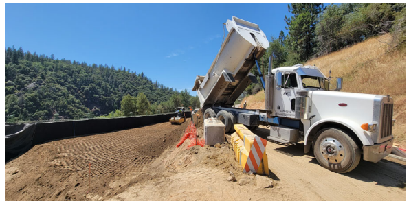
8/02/23 — Abutment 4 RW 4 Structure Backfill
