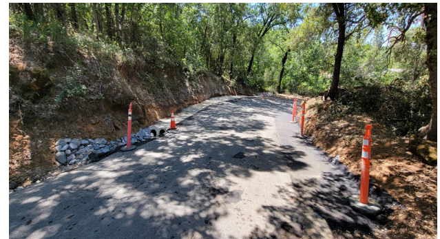
6/29/23 – South Switchback Improvements
