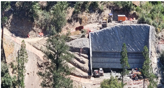
8/02/23 — Pier 2 Row 11-6 Architectural Concrete
