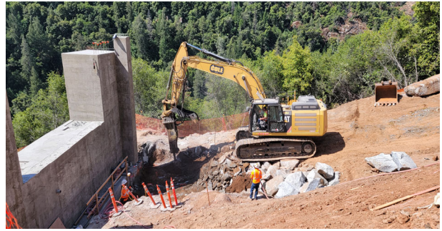
6/02/23 — Abutment 4 RW 4 Stage 1 Footing Rock
