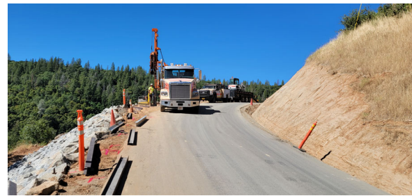
7/31/23 – North Metal Guardrail Installation
