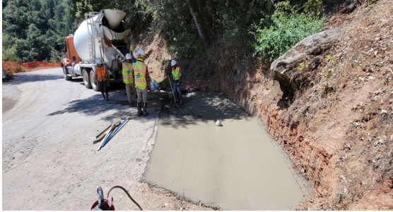
7/06/23 – Drainage System #5 Outfall Concrete Pour
