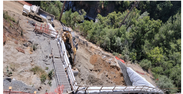
8/04/23 — Pier 3 Row 3 Post Blast Rock Excavation
