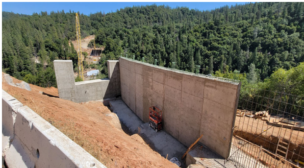
6/29/23 – Abutment 4 RW 4 Stage 1 Stem Forms Stripped
