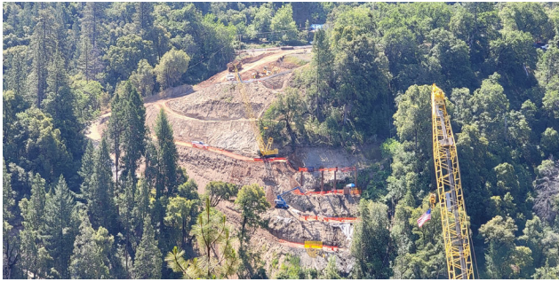
6/02/23 — Pier 2 Temporary Trestle Construction Excavation
