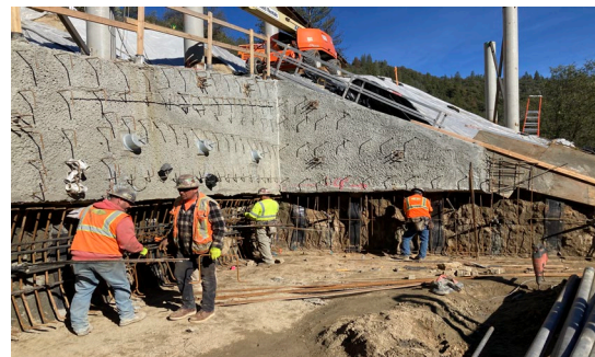
1/23/23 - Pier 3 Row 11 RW Placed Structural Rebar
