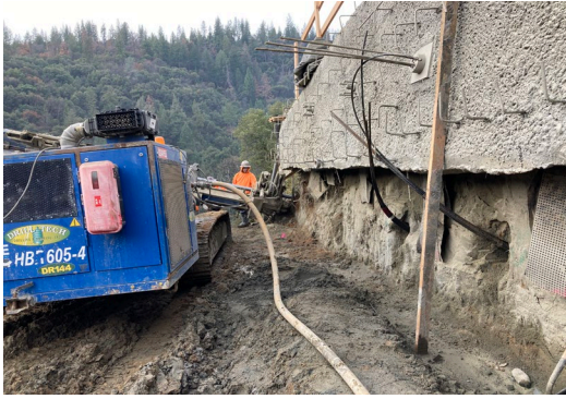
12/21/22 - Pier 3 Row 11 RW Anchor Drilling
