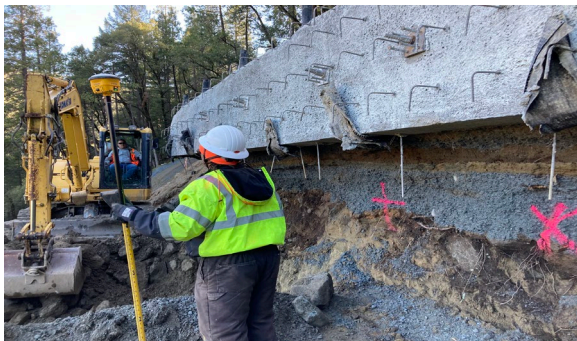
2/14/23 — Pier 2 Row 10 RW Structure Excavation
