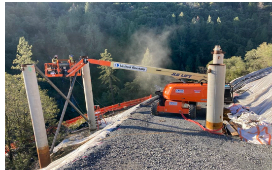
1/20/23 - Pier 3 Trestle Bracing Installation
