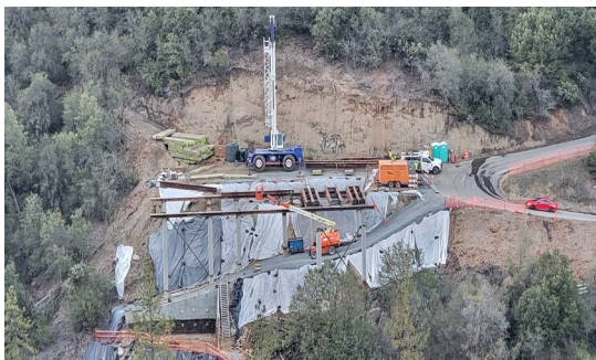
1/23/23 - Pier 3 Trestle Began Decking
