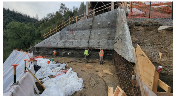
3/3/23 - Pier 3 Row 9 Shotcrete Placement
