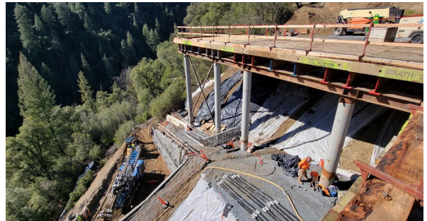
2/6/23 - Pier 3 Row 10 RW Structure Excavation
