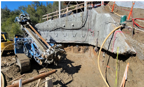
2/6/23 - Pier 3 Row 10 RW Structure Excavation
