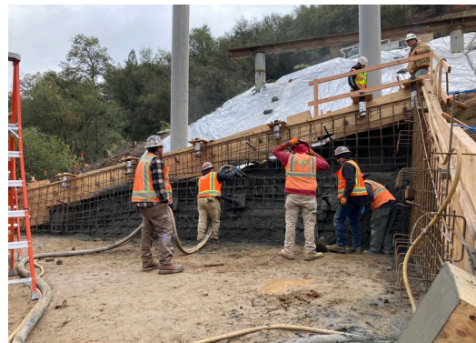
12/9/22 - Pier 3 Rows 13 & 12 Trestle RW Shotcrete
