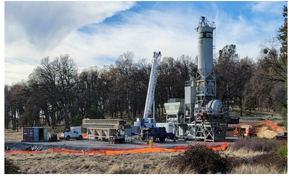
12/23/22 - Batch Plant Equipment Mobilization Complete
