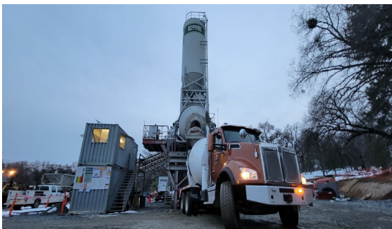
3/3/23 - Batch Plant Production for Pier 3 Shotcrete
