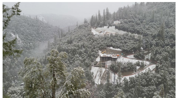
2/24/23 - Pier 3 Row 9 / Snow on Site
