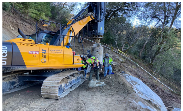
2/13/23 - Pier 2 Trestle Foundation Drilling
