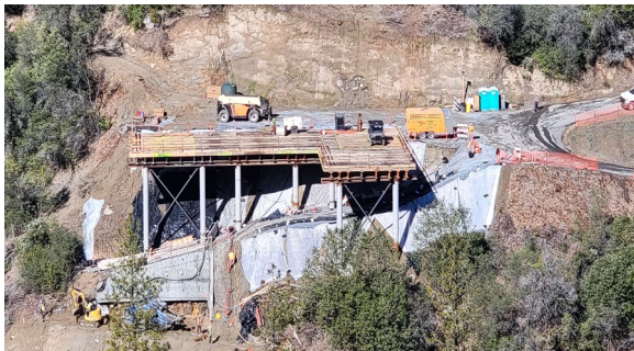
2/6/23 - Pier 3 Trestle Decking and Handrails Complete
