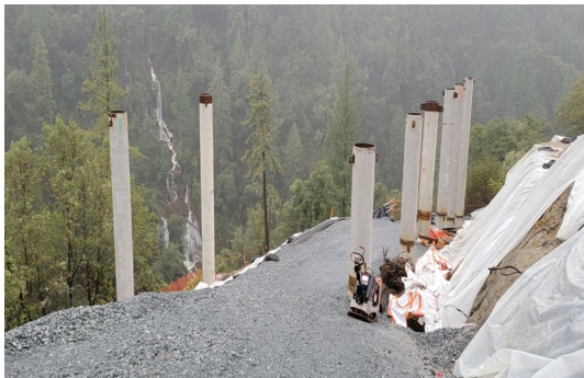
1/9/23 - Pier 3 Trestle Prior to Decking – Rain Day
