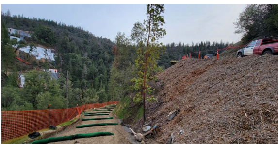
3/3/23 — Pier 3 Access Erosion Control Maintenance
