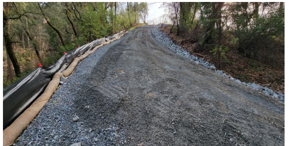
3/3/23 - Pier 2 Access Erosion Control Maintenance
