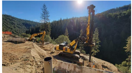
Pier 3 Trestle Pile Foundation Drilling
