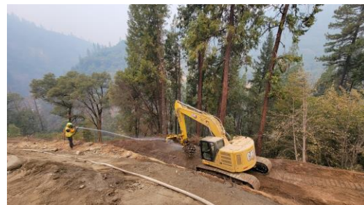
Pier 2 Trestle Drill Bench Grading
