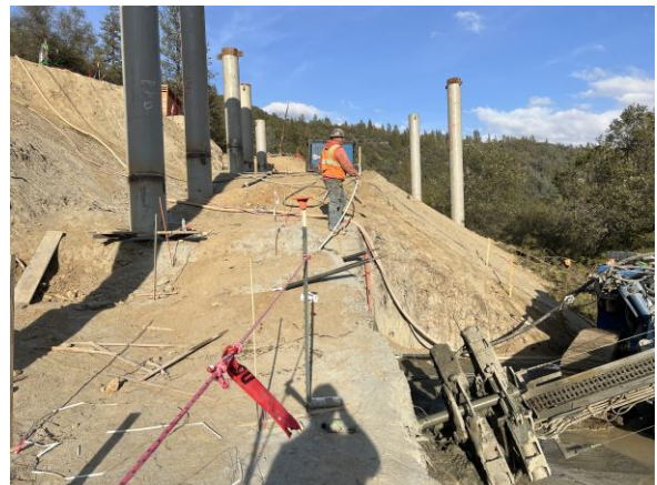
Pier 3 Trestle Pile Foundation / Ground Anchor Drilling
