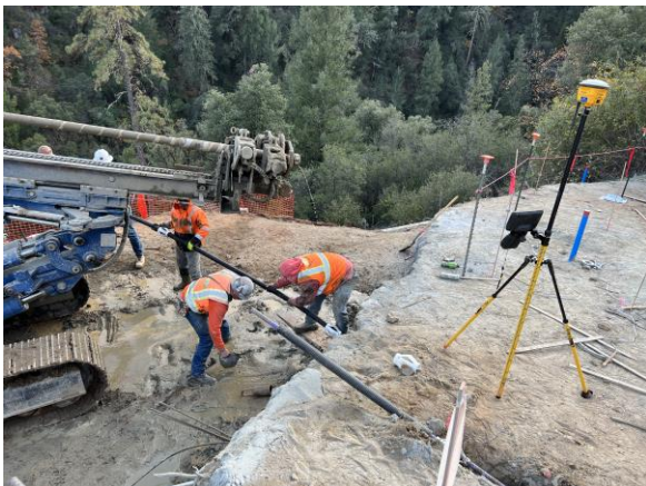
Pier 3 Ground Anchor Installation
