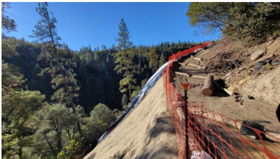
Pier 3 Access Road and Erosion Control
