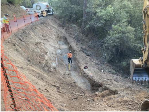
Pier 3 Access Retaining Wall Construction
