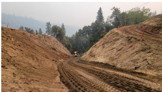
South Approach / DS 3 Embankment Preparation
