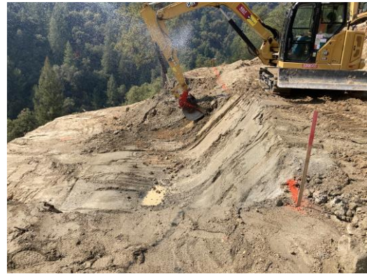
Grading for Pier 3 Trestle Foundation Drilling Tables
