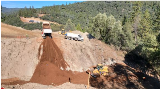
South Approach / DS 3 Embankment Fill Progress
