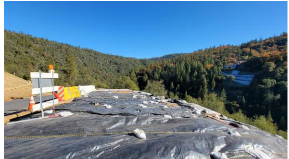
Site Wide Erosion Control Measures
