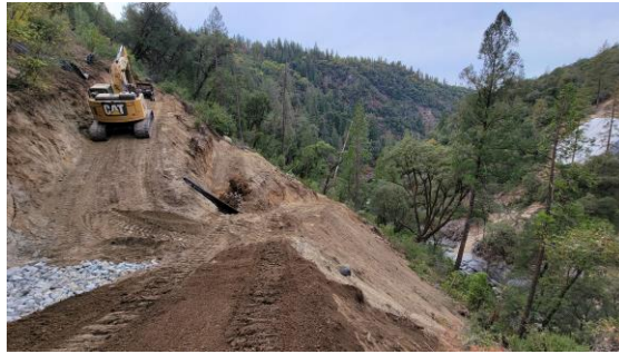
Pier 2 Ground Anchor / Soil Nail Retaining Wall Access
