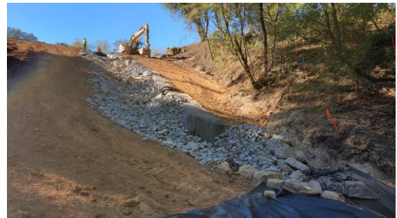
DS 3 Outfall Rock Armoring Progress
