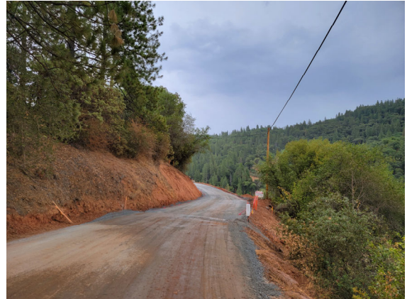
North Road Realignment
