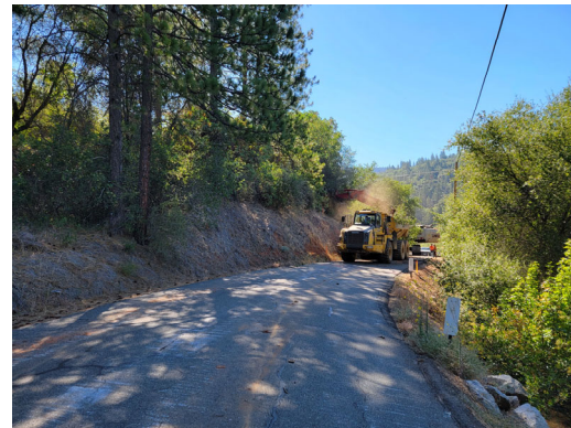
Existing North Road
