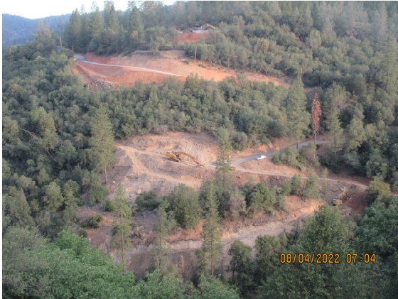
View from South Abutment 1 towards North Abutment 4
