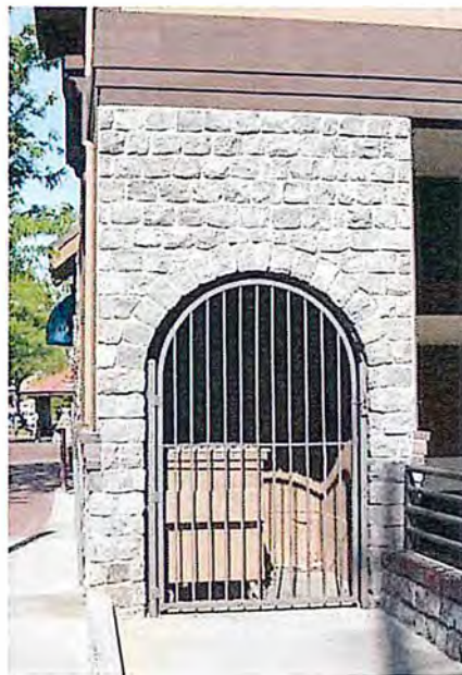
Utilities should be screened with landscaping
