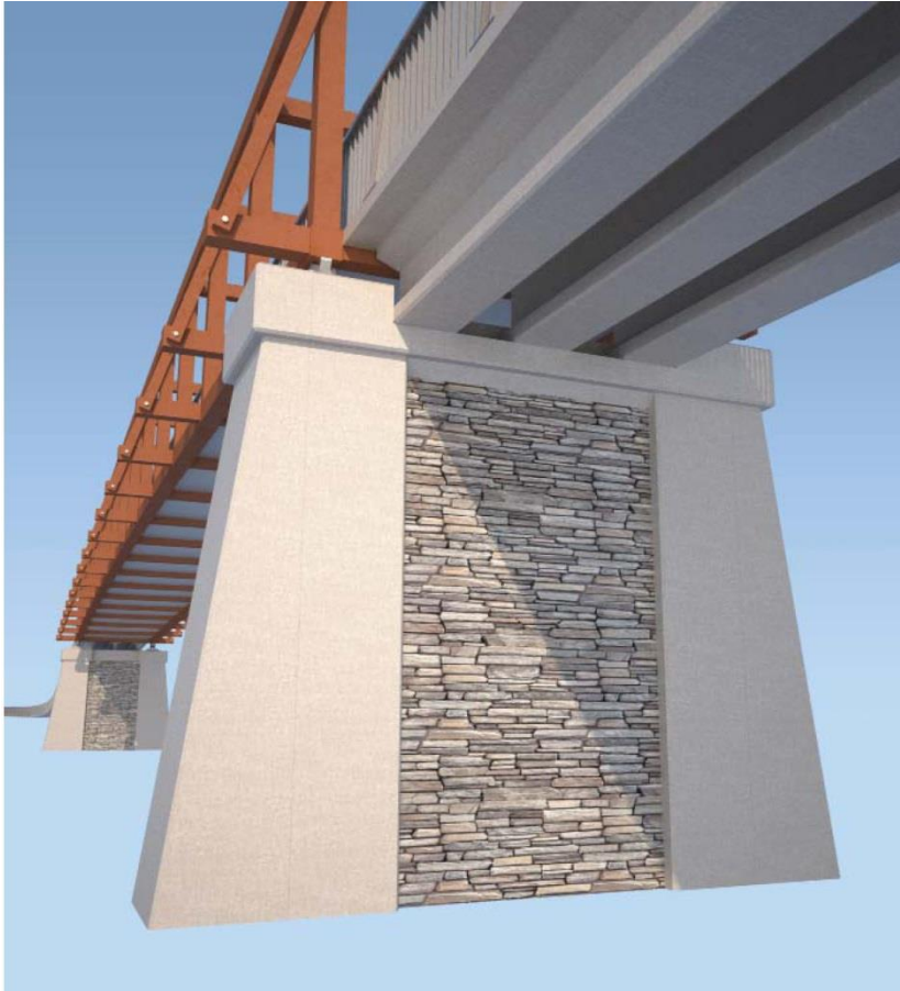
Stacked Rock & Concrete Pier
