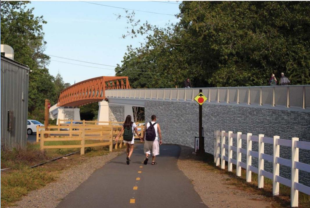
Stacked Rock Retaining Wall
