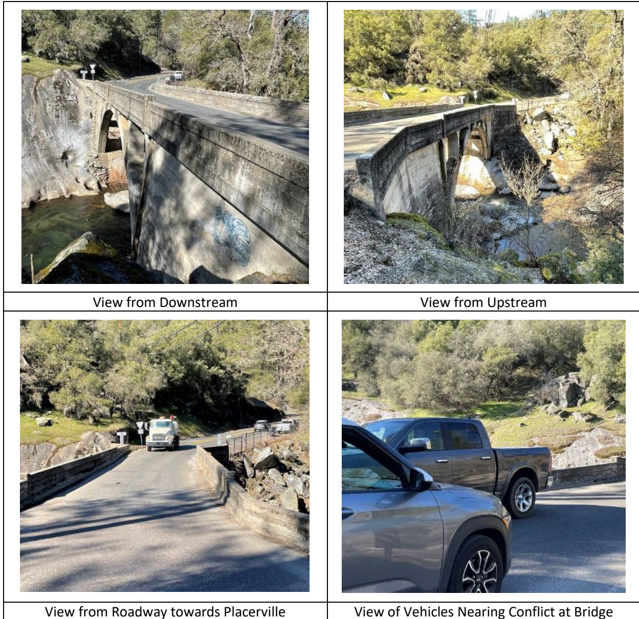
Exhibit 2-2 Bucks Bar Road Existing Bridge
