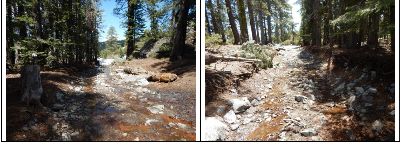
Walker Hill RT Station 170+80
