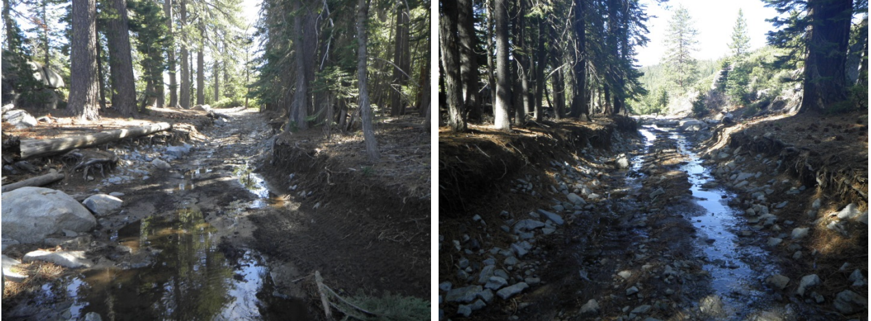
Walker Hill RT Station 170+80
